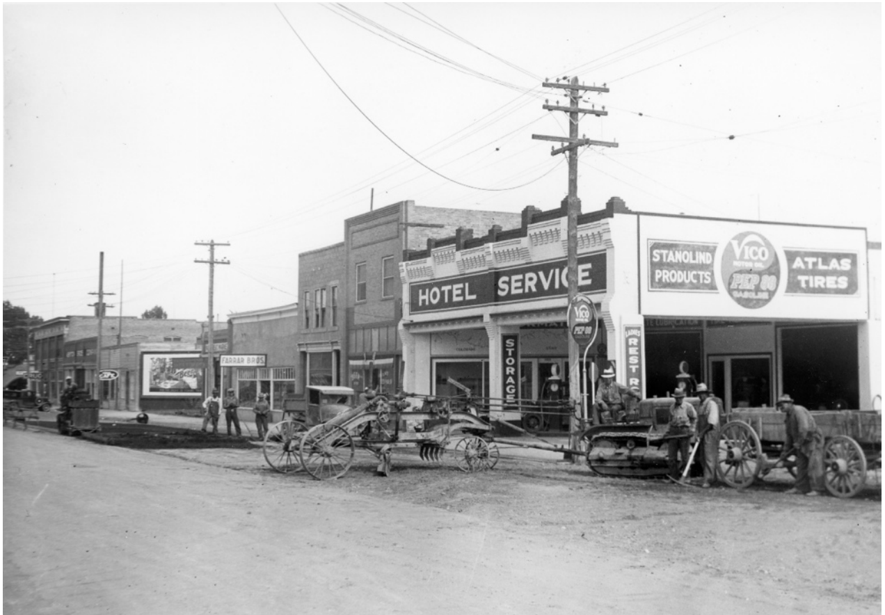
Figure 28. Photograph of Main St. paving, 1934. Credit: Leo Thorne. Source: Uintah County Library Regional History Center.
