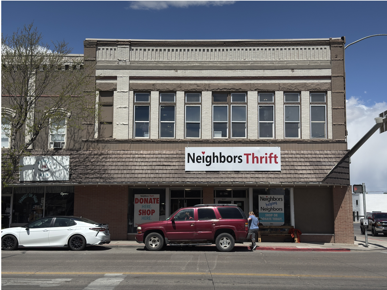
Figure 6. Photograph of the former Ashley Co-op building at 4 W. Main St., 2025. Credit: Kirk Huffaker Preservation Strategies.
