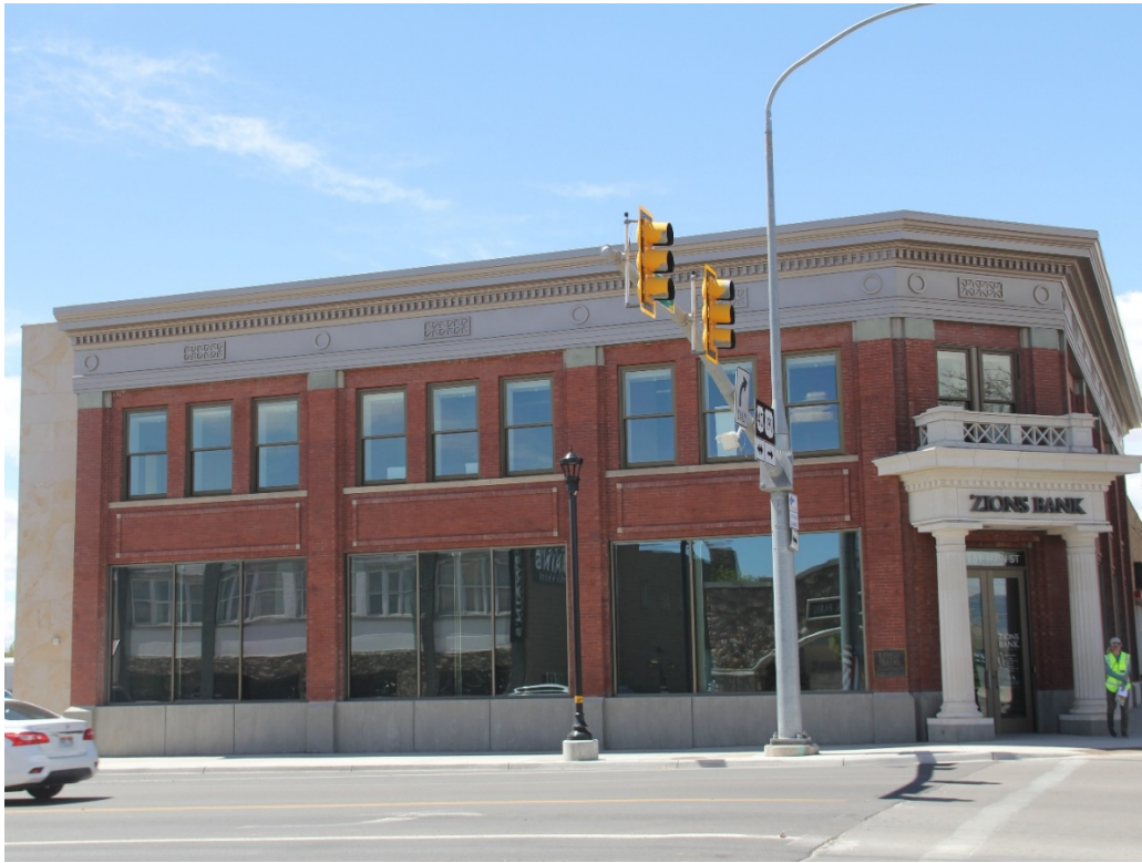
Figure 18. Photograph of the former Bank of Vernal building at 3 W. Main St., 2025. Credit: Kirk Huffaker Preservation Strategies.
