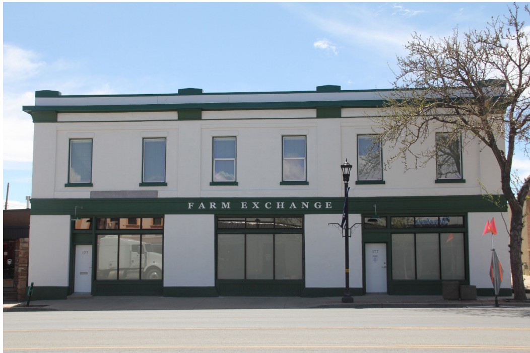
Figure 27. Photograph of the Farm Exchange Building at 177 W. Main St., 2025. Credit: Kirk Huffaker Preservation Strategies.
