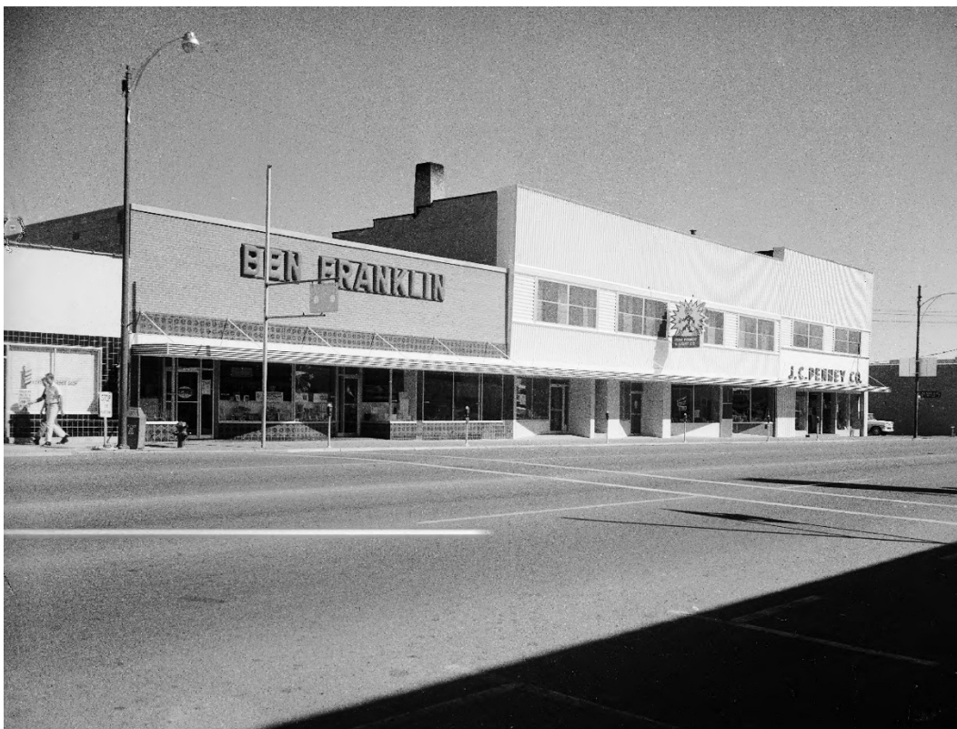
Figure 5. Photograph of the Ashley Co-op Building, 1962. Credit: Leo Thorne. Source: Utah State Historical Society.
