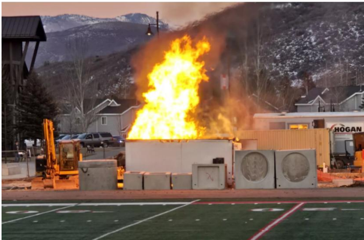
PCHS Construction Trailer Fire
