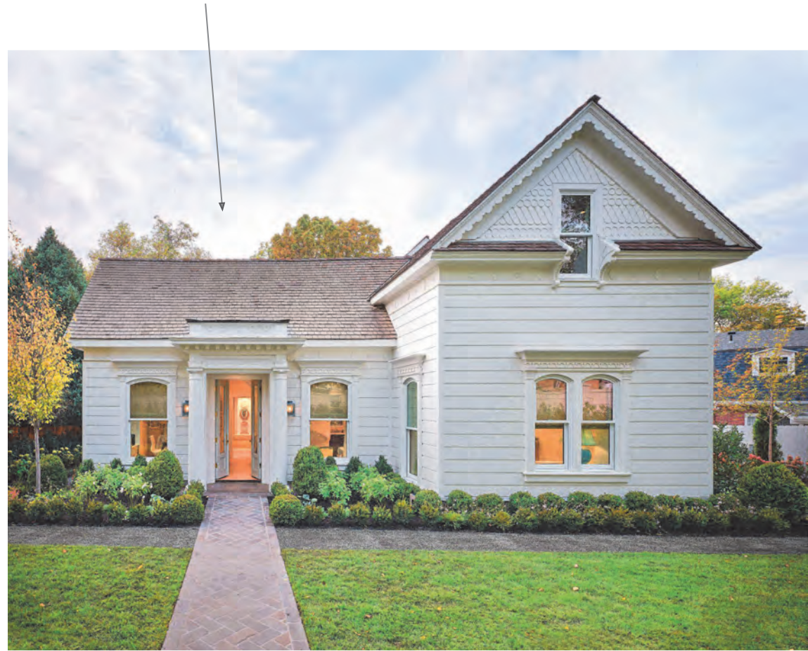
Replacement windows mimic 1870-90 late victorian
