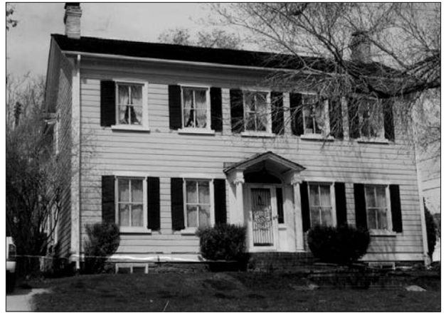
Classical Porch, at central entry.
