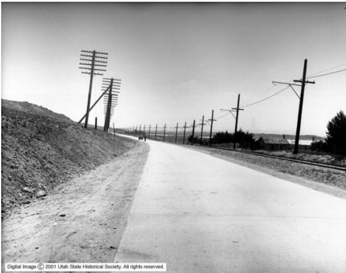
Highway 89 Beck Street
