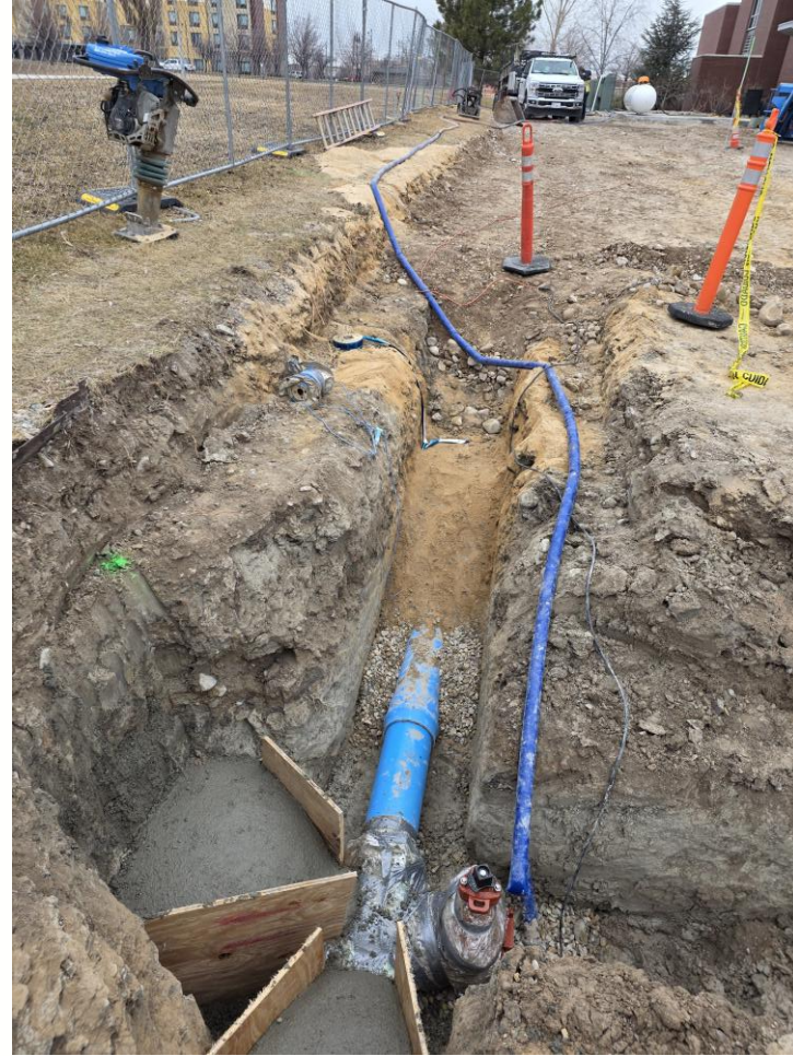
6" fire line and thrust blocks
