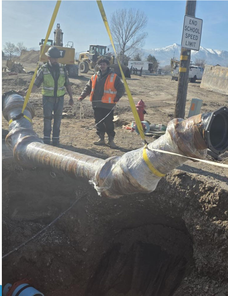
12" ductile iron water line loop
