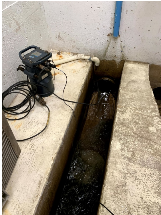
Figure 2-7: Typical Submerged AV Installation (Influent to 2280 Lift Station)
