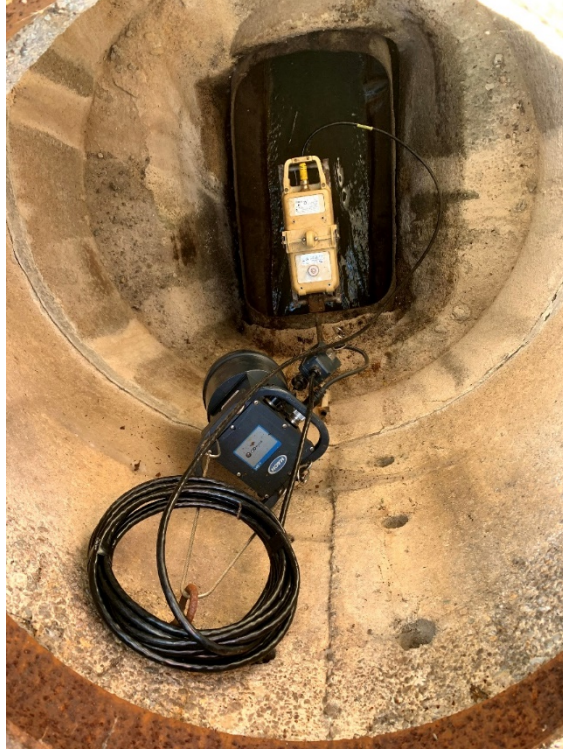
Figure 2-6: Typical FLO-DAR Installation (MH-W11)
