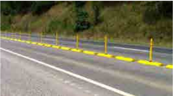
Flexible delineator with rubber curb
