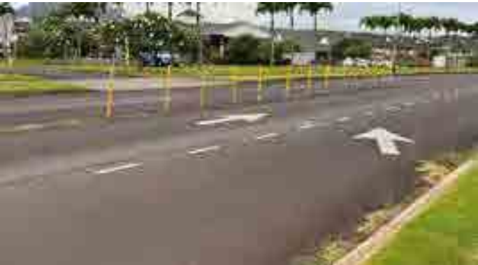
Flexible delineator with rubber curb
