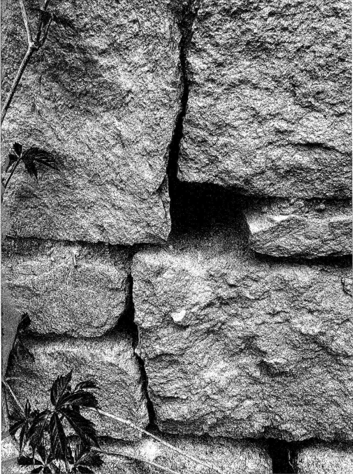
Deteriorated Mortar
