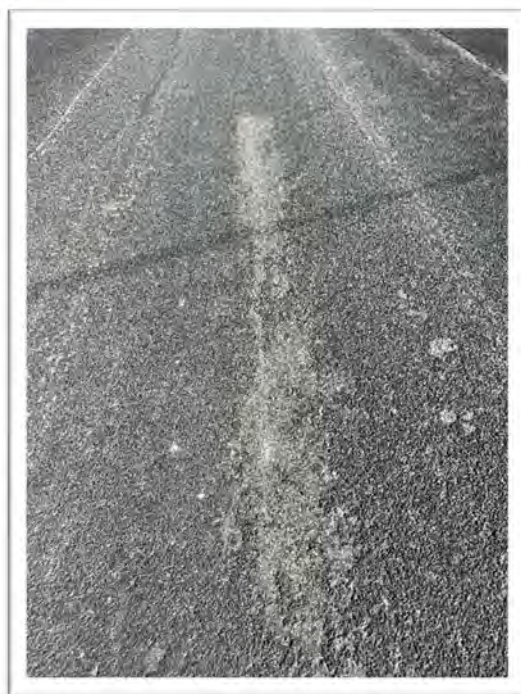
Exhibit 9 – Chip Seal Treatment Degradation
