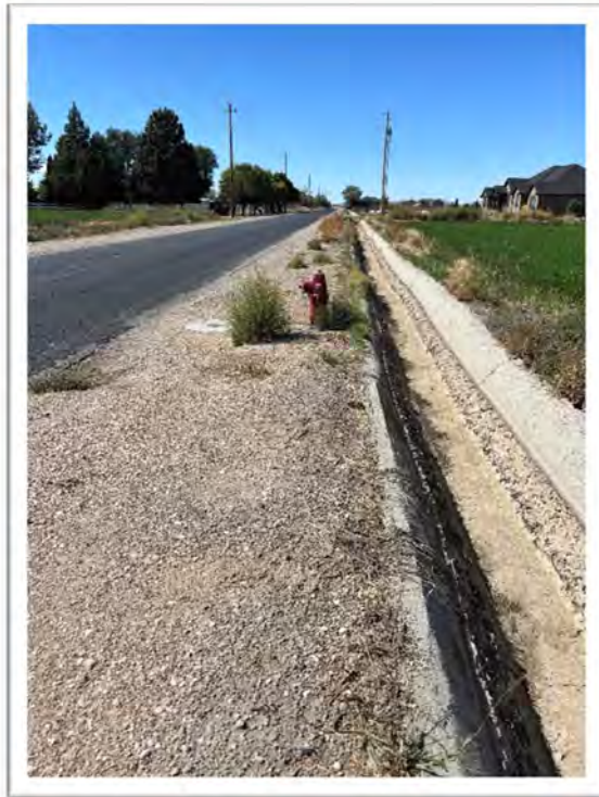
Exhibit 15: Lined Open Ditch on North Side
