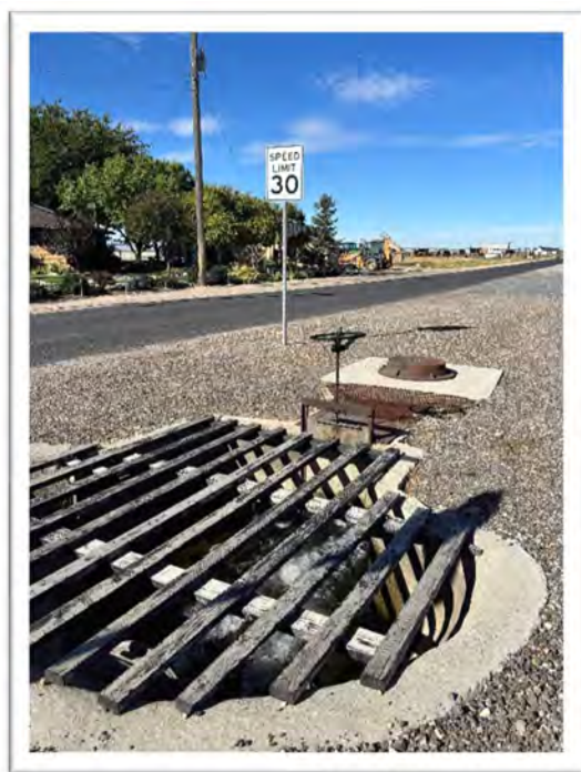
Exhibit 12 – Structure with Wooden Grate
