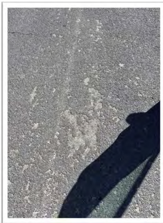
Exhibit 5 – Deterioration of Chip Seal Treatment
