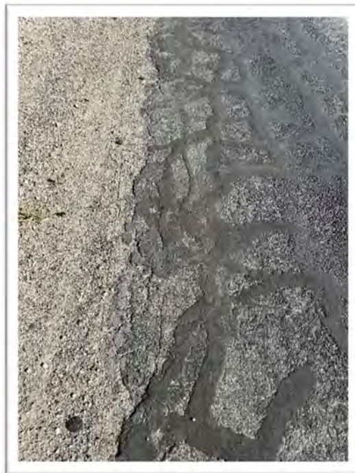
Exhibit 8 – Additional Fatigue Crack Sealing on Road Edge
