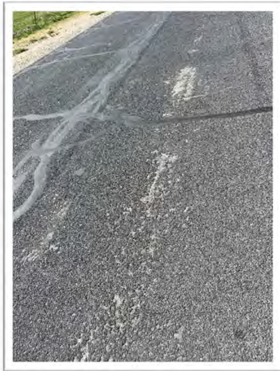
Exhibit 19: Chip Seal Treatment Degradation on West End
