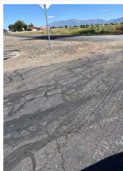
Exhibit 3 – Fatigue Crack Sealing with Recent Cracks Visible
