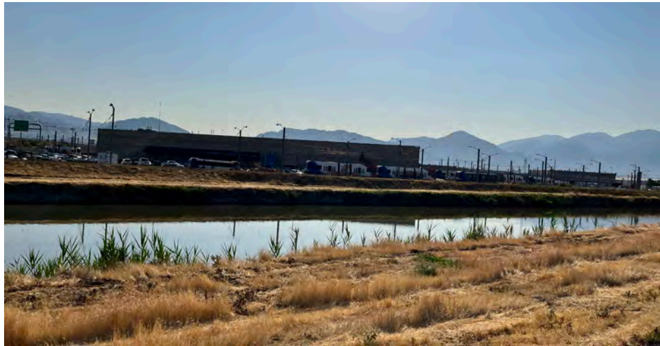
VEGETATION ALONG THE FEDERALLY REGULATED LEVEES HAS TO BE FREQUENTLY MOWN TO ABIDE BY ARMY CORPS REGULATIONS.
