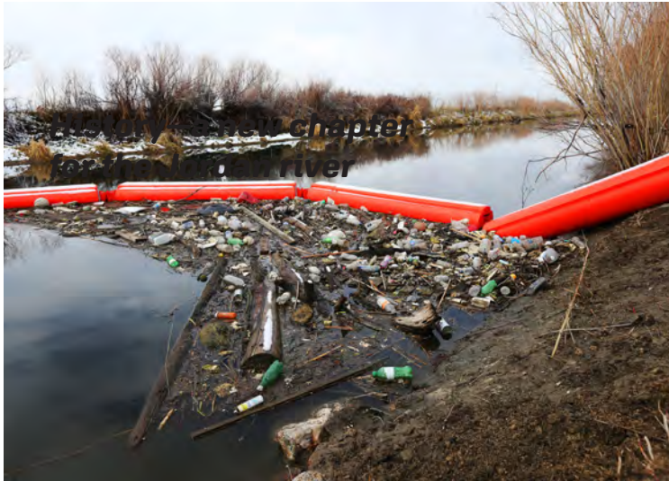
A trash boom in Jordan River traps floating garbage in an effort to protect Great Salt Lake wetlands and waterfowl. https://www.ksl.com/article/46298298/jordan-river-trash-boom-targets-floating-garbage-protects-great-salt-lake-wetlands
