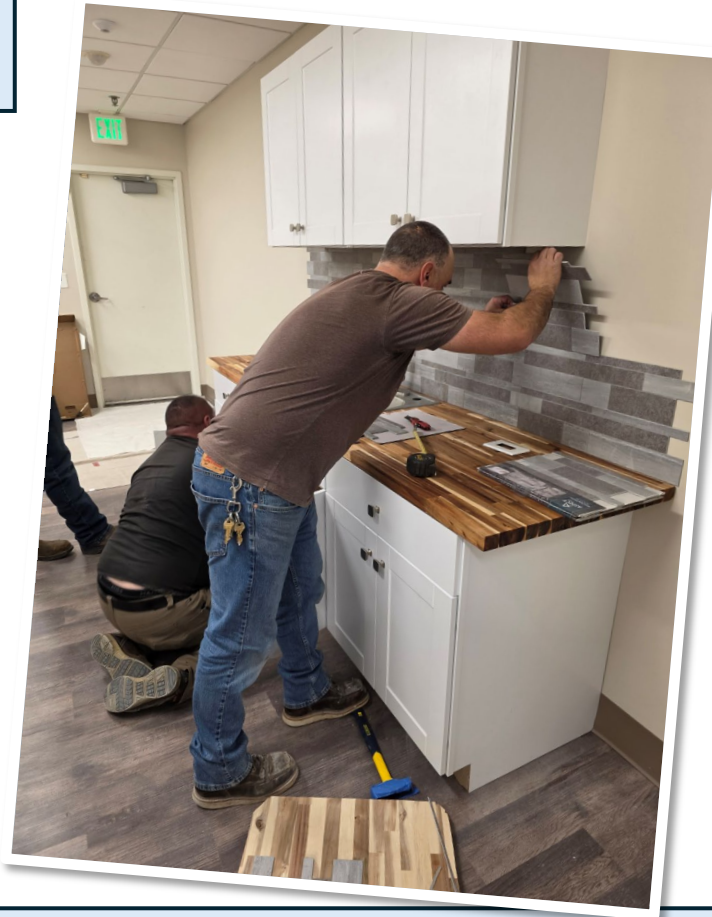
The operations team remodeling and installing a kitchen counter in building A basement.
