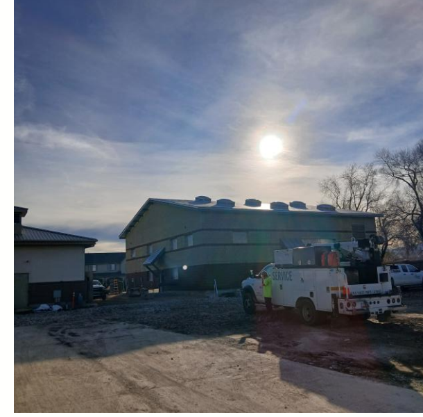
Anderson WTP – Roof installation
