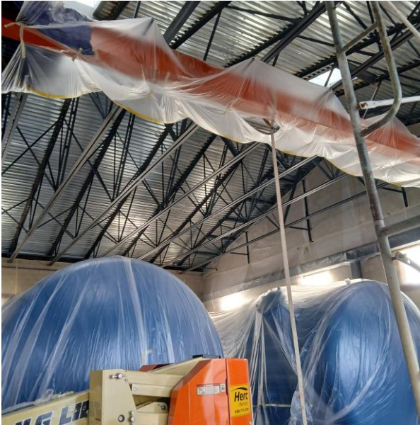
Anderson WTP – Interior prepped for painting
