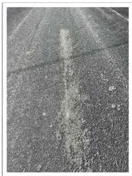
Exhibit 9 – Chip Seal Treatment Degradation
