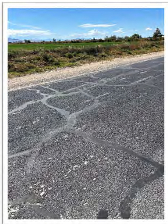
Exhibit 18: Fatigue Cracking on West End
