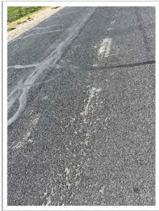
Exhibit 19: Chip Seal Treatment Degradation on West End
