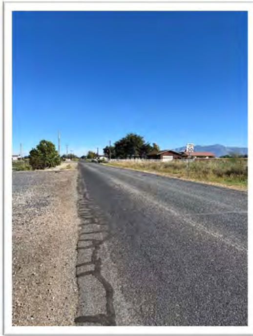
Exhibit 7 – Fatigue Crack Sealing on Road Edge
