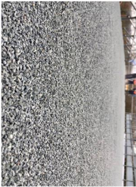
BALLASTED FLAT ROOFS
