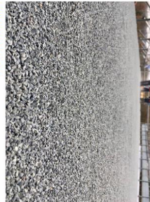
BALLASTED FLAT ROOFS
