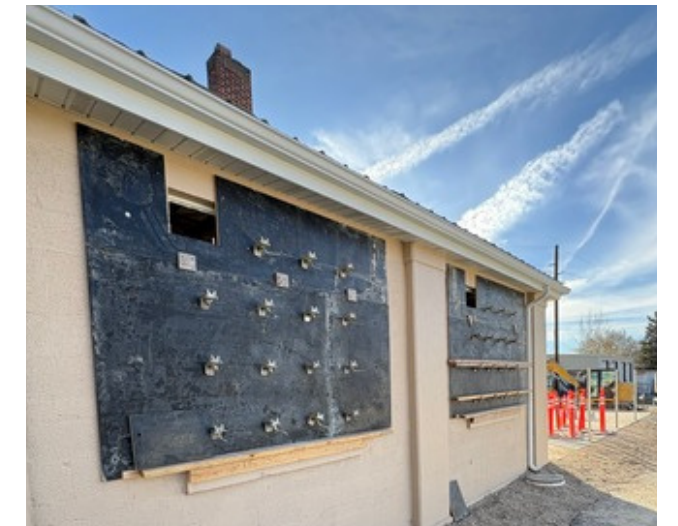
11/11/25 Windows being blocked in with concrete.
