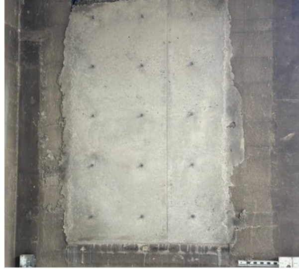
Shown here window blocked in. 1 of 8 windows
