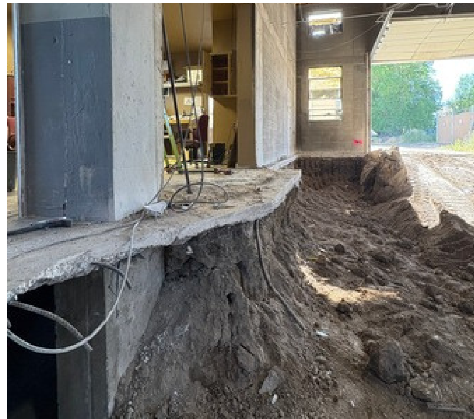
Concrete all removed from building
