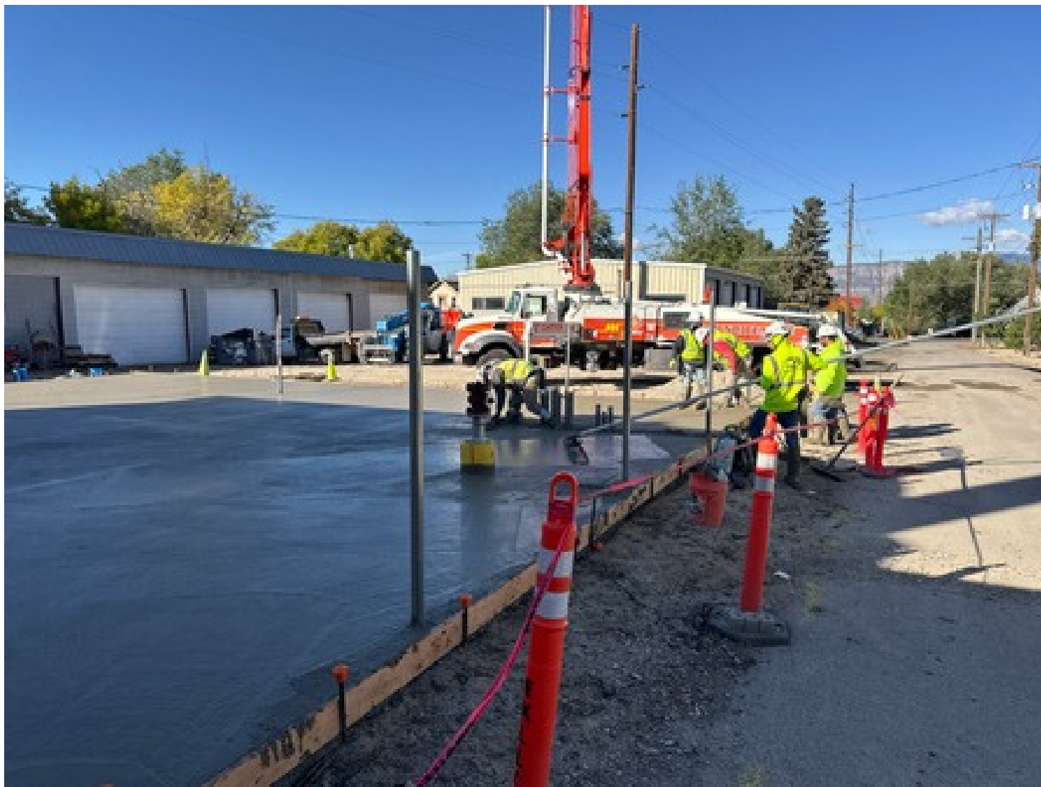
Radiator,Oxy catalyst pad being poured 10/6/25
