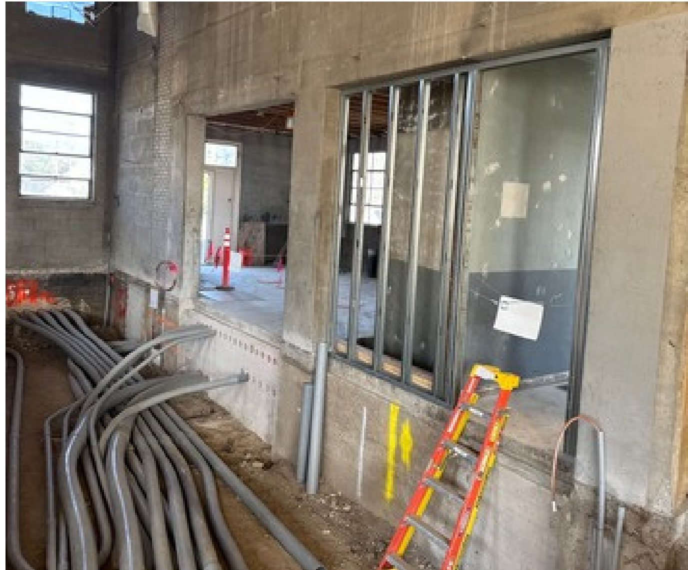
Start of main conduit install 9/29/25
