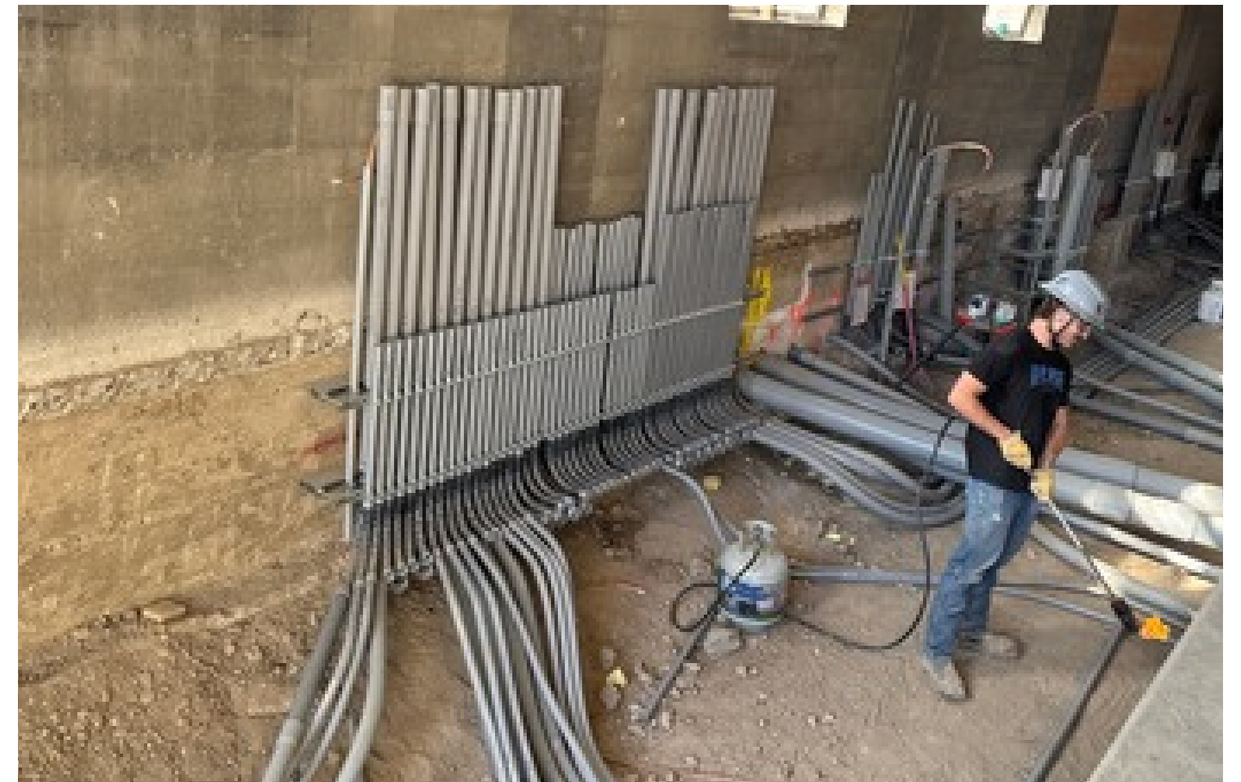
Conduits being heated to be bent for placement 9/29/25
