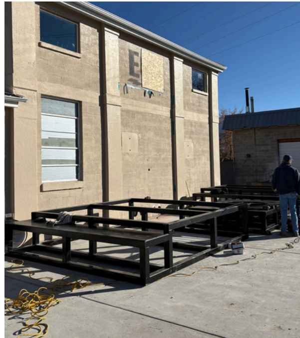
Stand installed for swamp cooler and OXY catalyst stack
