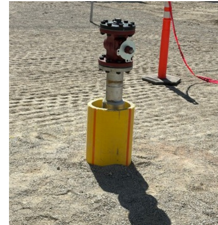
4" Gas stub installed 9/17/25
