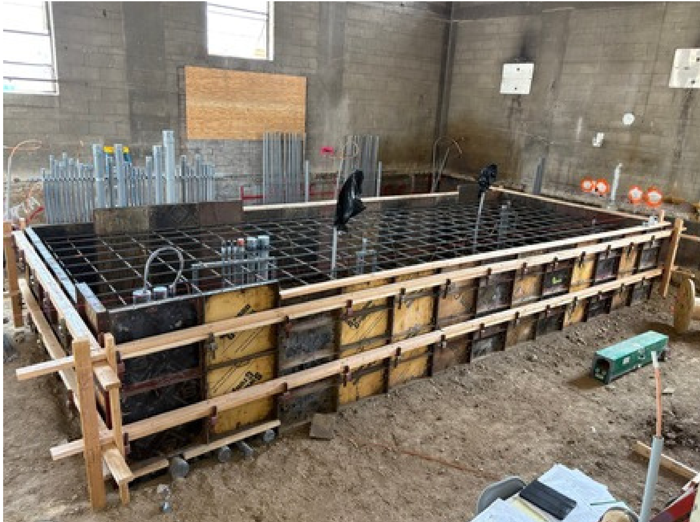
First generator pad ready for concrete
