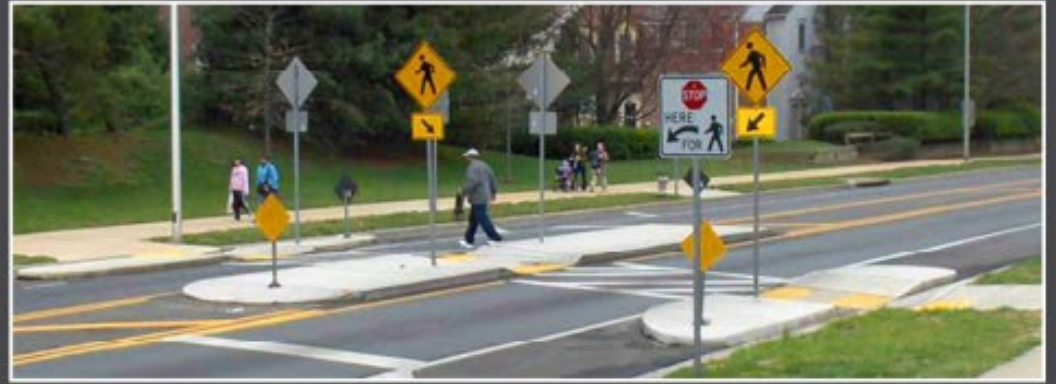
MID-BLOCK CROSSING WITH CENTER PEDESTRIAN REFUGE
