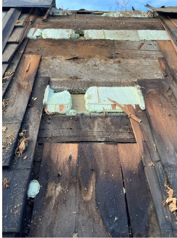
Figure 1- Deterioration at Ridge Boards
