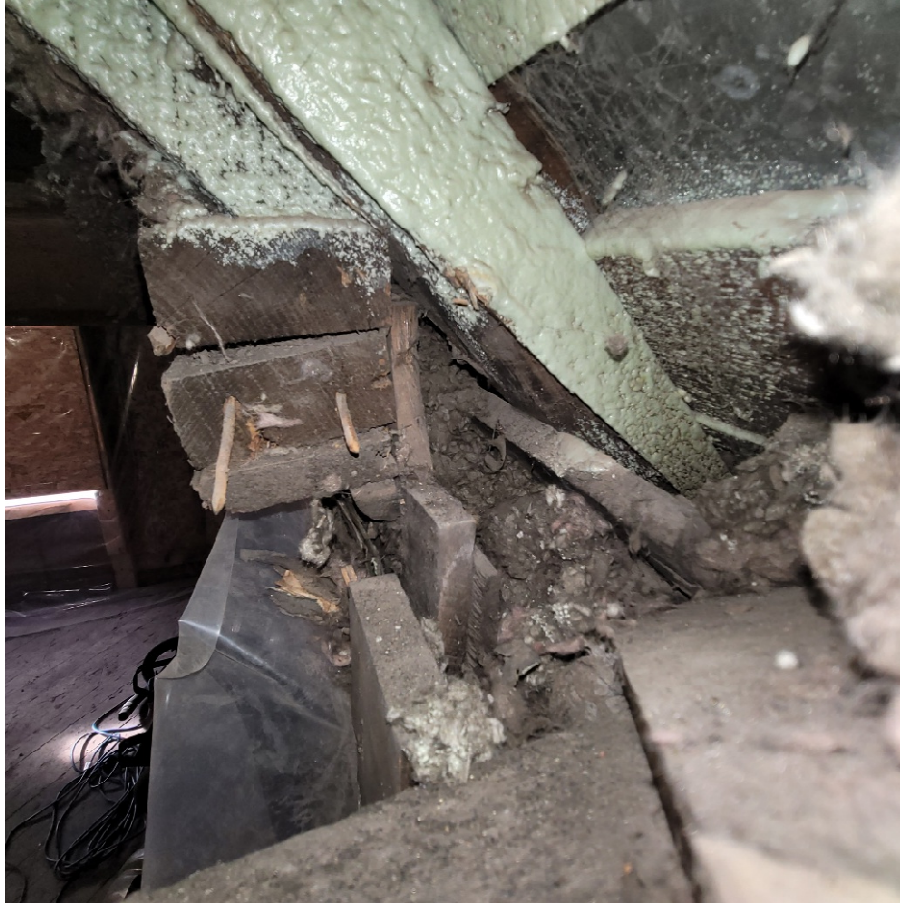
Figure 5 - Improper Framing Example 3, Including Deterioration
