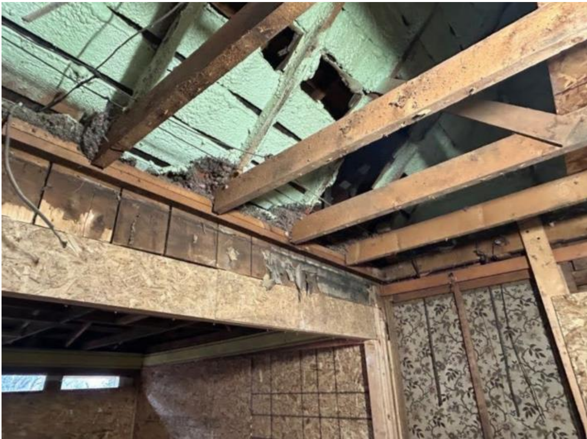
Figure 2: Applicant's photo showing deteriorated roof structure on the Significant Historic Structure at 218 Sandridge Road in October 2025.
