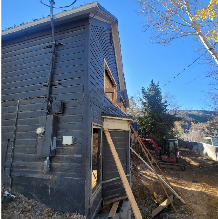
Figure 7 - Bowing of Wall
