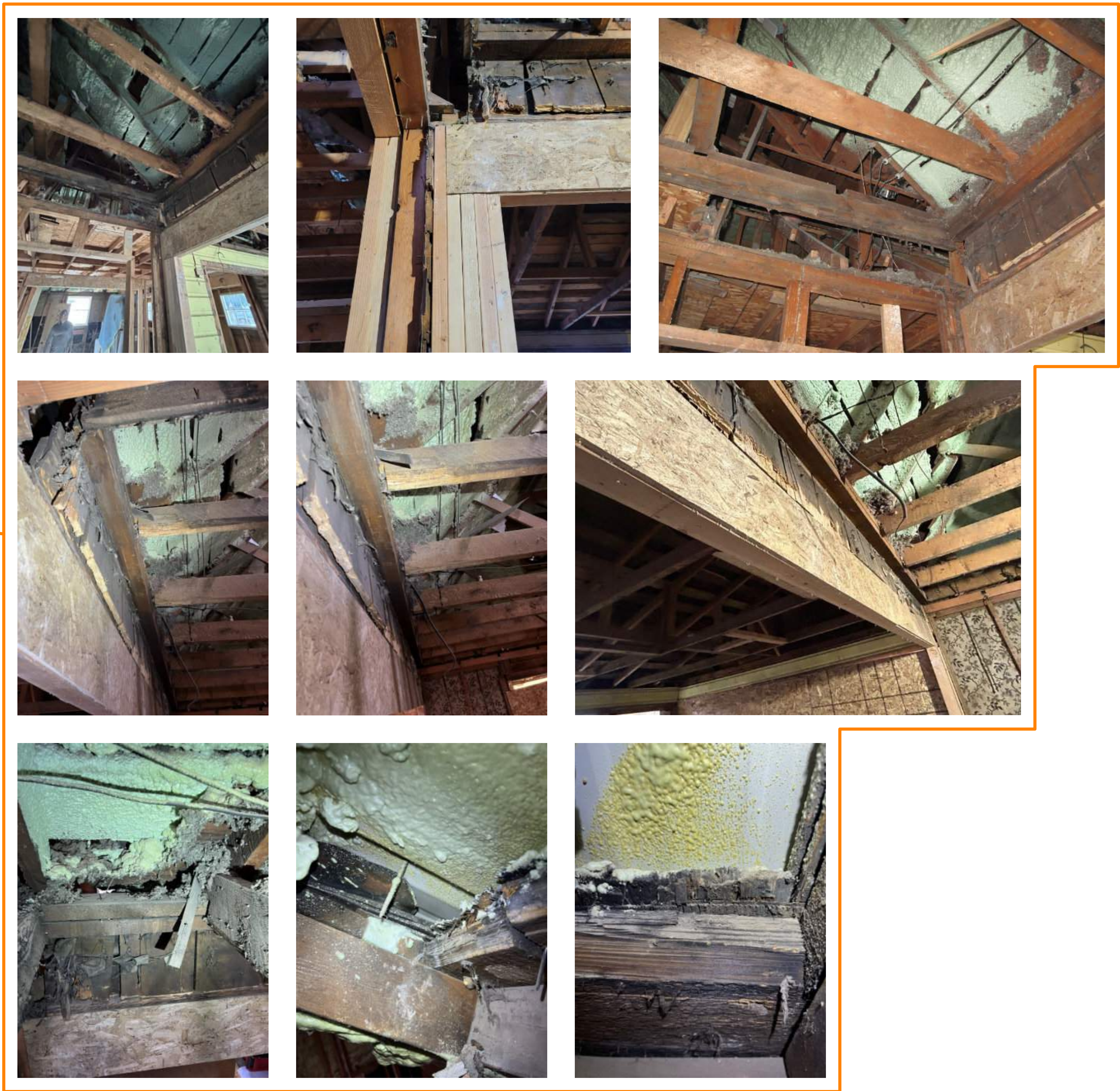
Advanced rotting paired with improper framing
