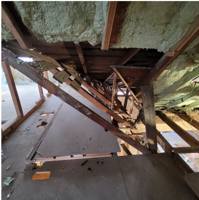
Figure 4 - Improper Framing Example 2
