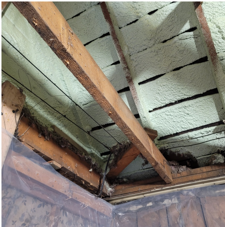
Figure 8 - Notched Ceiling Joists
