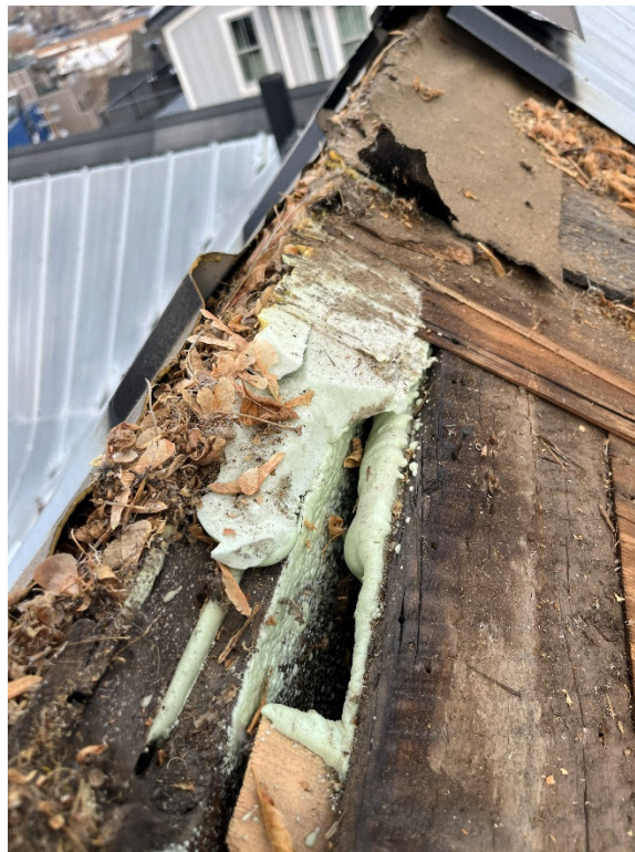
Figure 2 - Deterioration of Ridge Board
