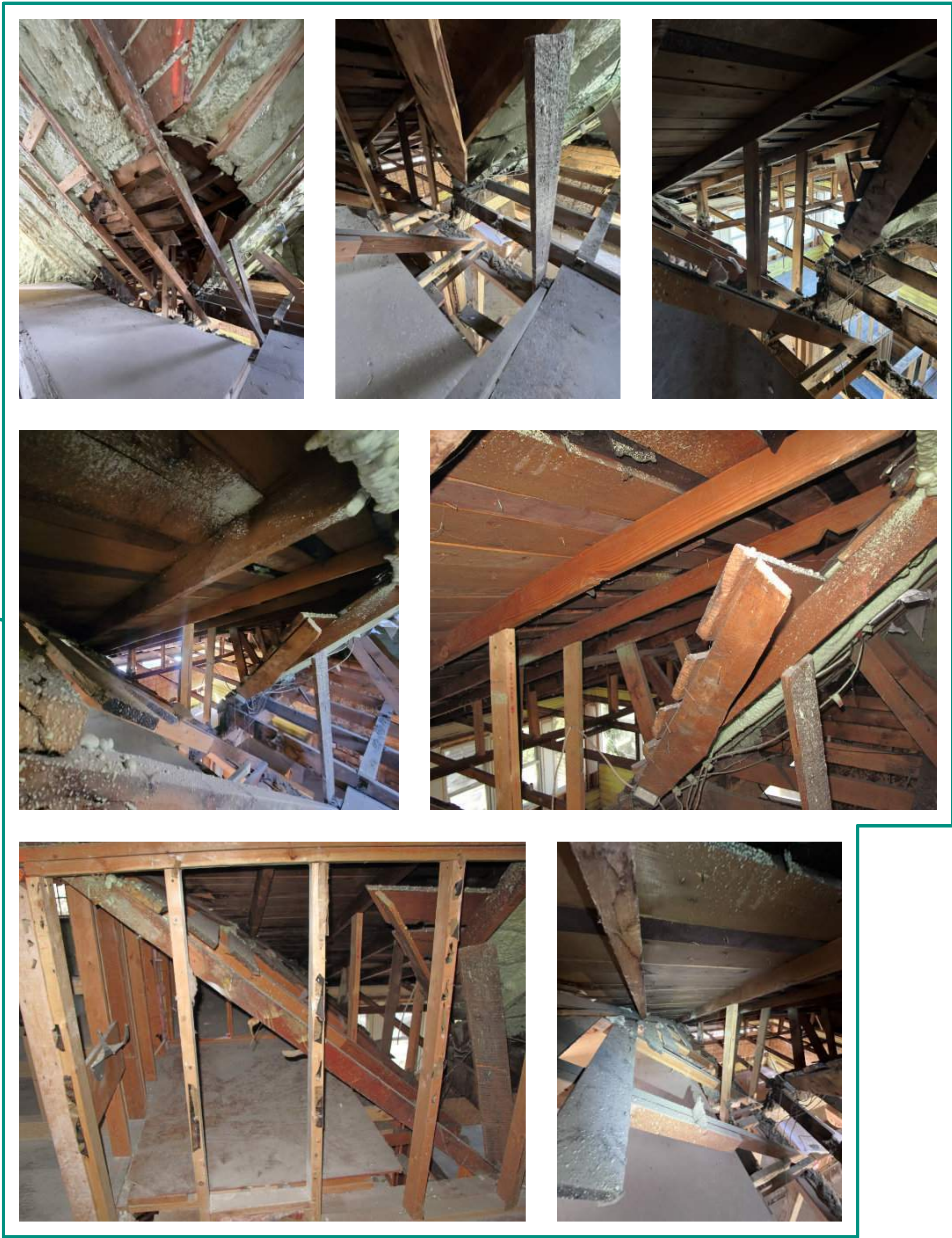
Incomplete and improper framing
