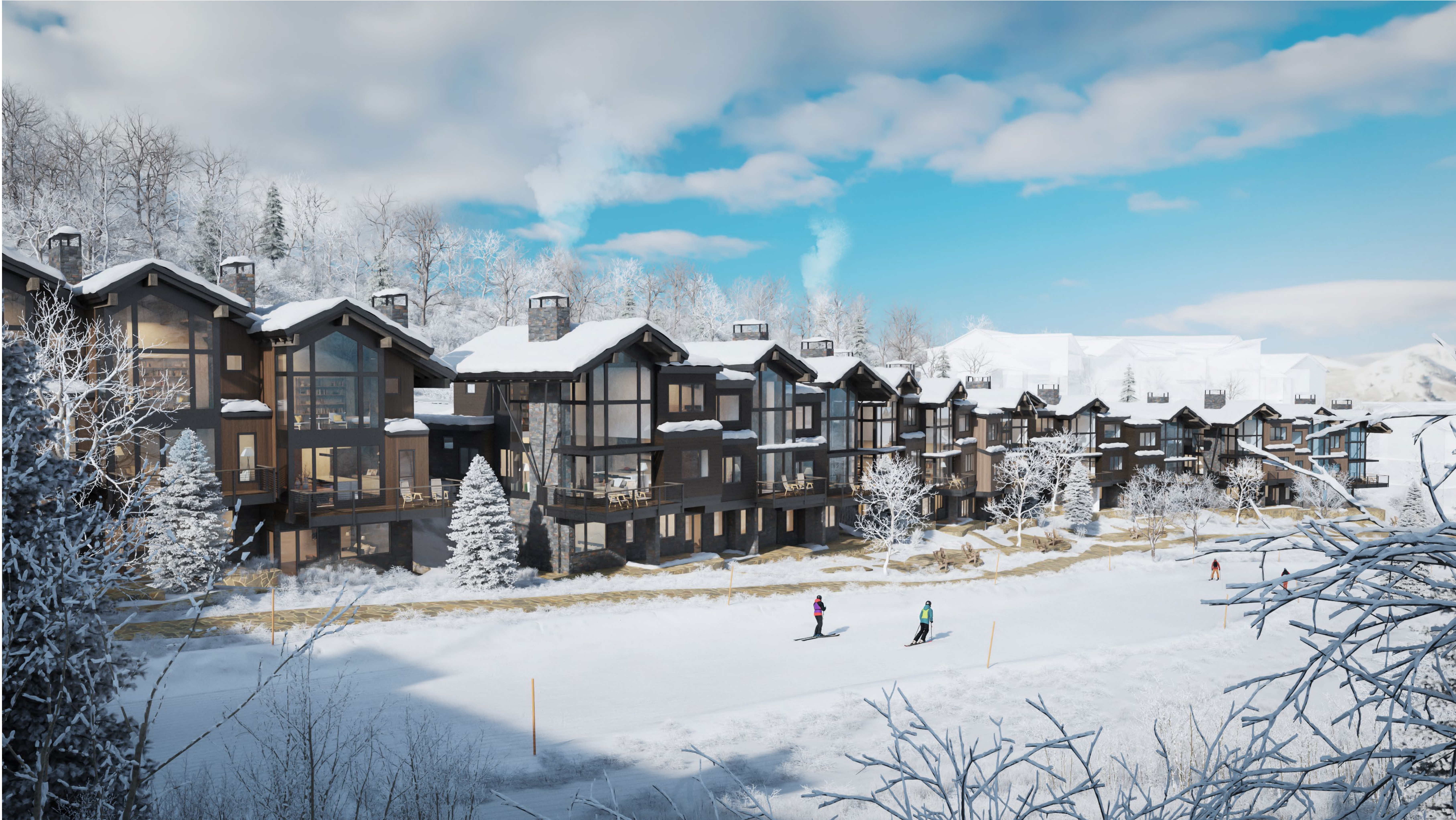
GROUND VIEW FROM BRIDGE
