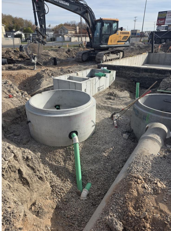
1,000-gallon grease interceptor and sample manhole
