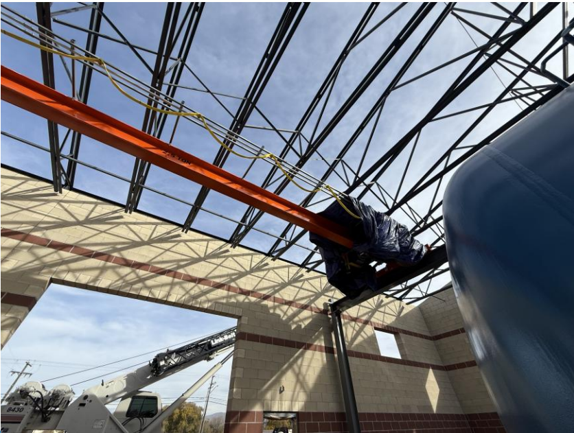
Anderson WTP - Overhead Crane Monorail and Roof Trusses
