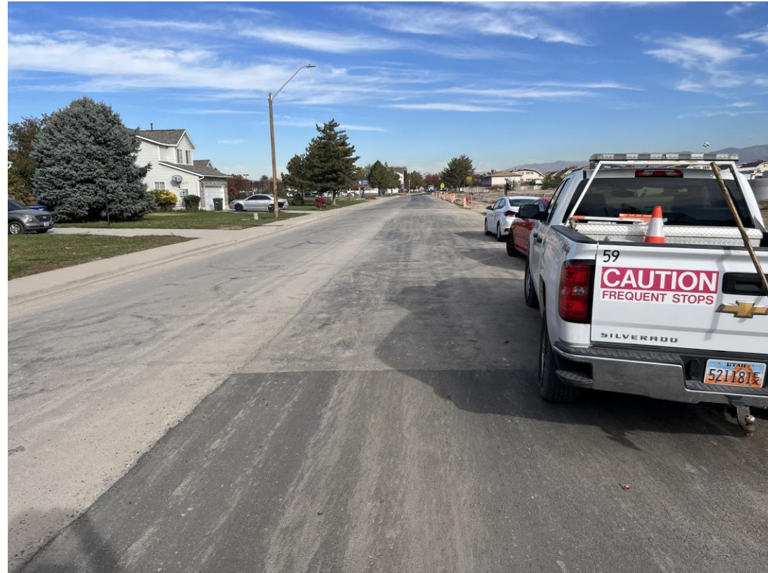
1950 W – Final Paving Prior to Raising Manholes to Grade
