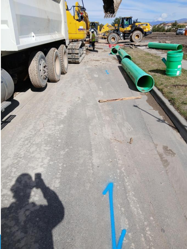
1950 W – Sewer Main Installation along the southern side of 1950
