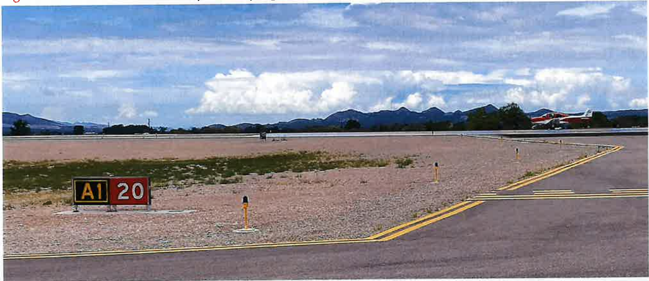
Figure 4.14: Medium Intensity Taxiway Lights
