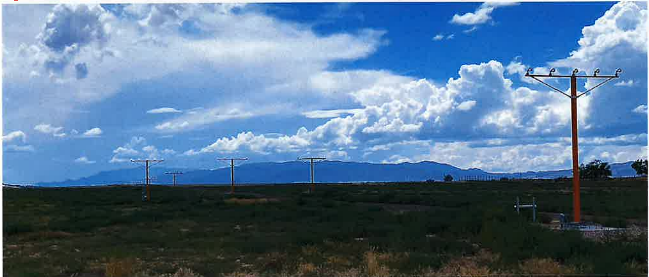
Figure 4.11: Medium Intensity Approach Lighting System with Runway Alignment Indicator Lights
