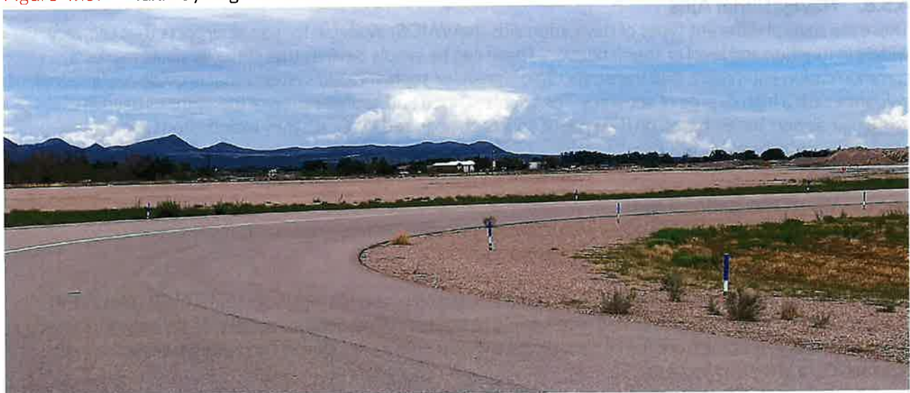
Figure 4.15: Taxiway Edge Reflectors
