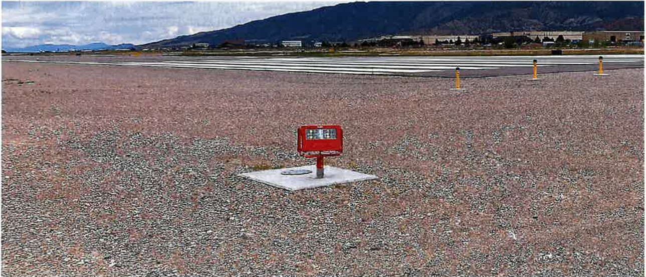
Figure 4.12: Runway End Identifier Lights
