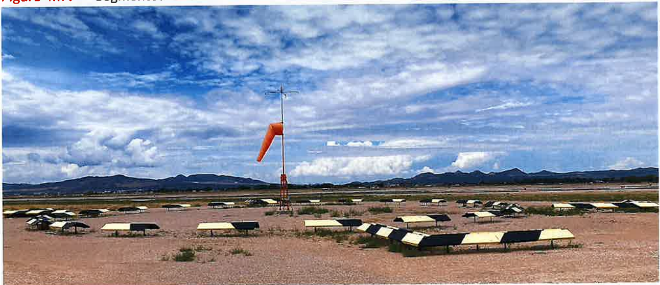
Figure 4.17: Segmented Circle and Wind Indicator
