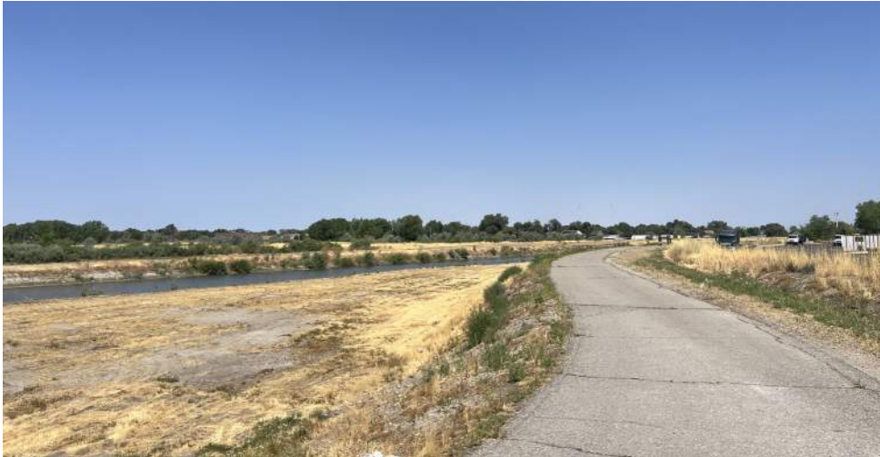
THE 10-FOOT-WIDE JORDAN RIVER TRAIL ATOP THE LEVEES HAS FREQUENT CRACKS AND SCRUBBY VEGETATION ENCROACHING IN SOME SECTIONS.
