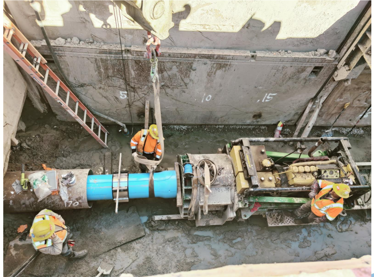
Well No. 18 Waterline – Bore Machine Installing Mainline Pipe
