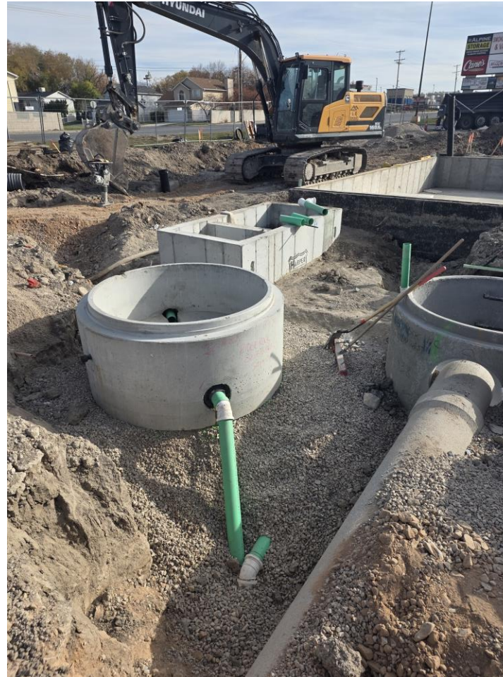
1,000-gallon grease interceptor and sample manhole
