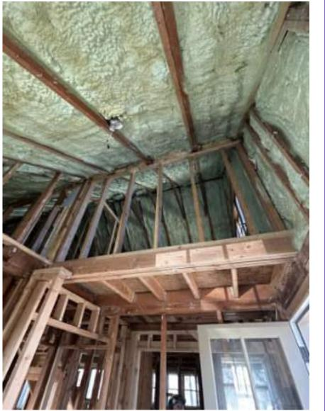
Corrugated metal roof is leaking, trapping moisture between original shingles and spray foam. Wood shingles and planks are rotten and very brittle.
