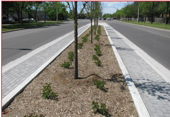
Stormwater management in the median underground bioretention.
