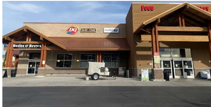
Required: Clearly identifiable covered entry
