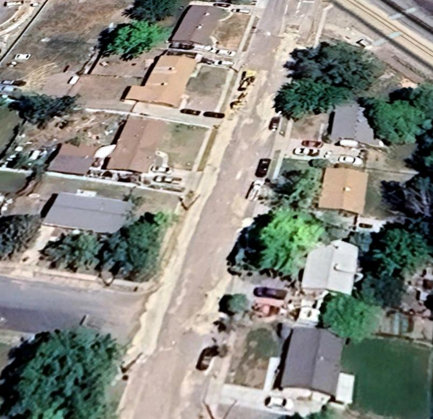
100 W After (5/2025 During Construction)
