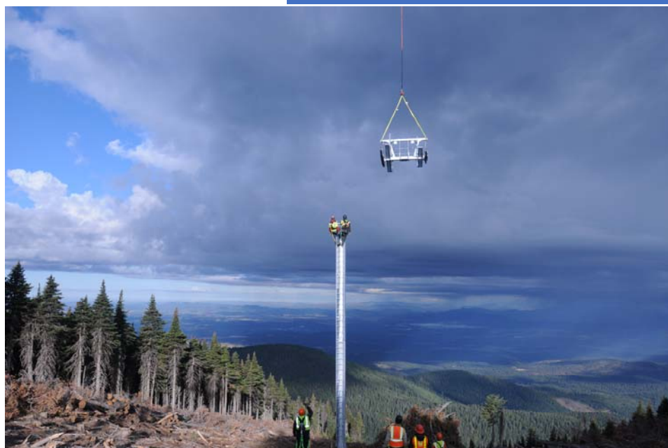
Picture #5 –Pole Construction
