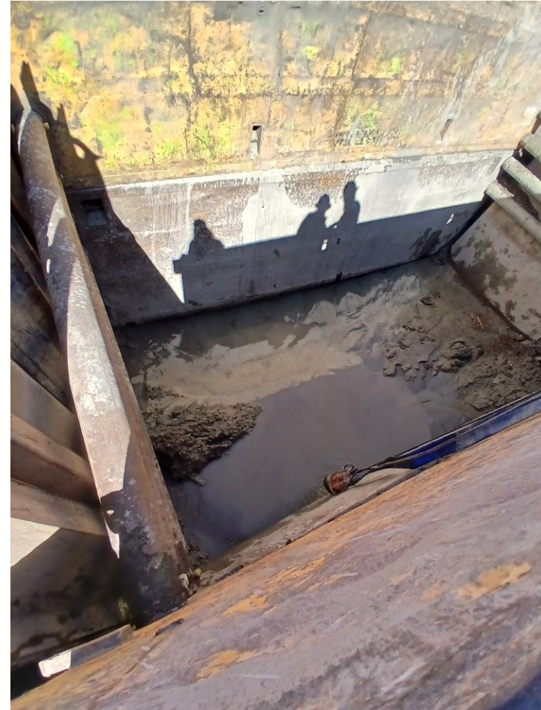
Collapsible Soil Material Below Water Table
