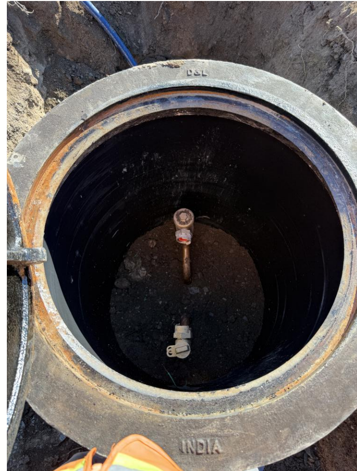
1" meter relocated out of sidewalk for new WVC park
