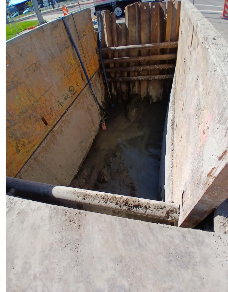
Well No. 18 Waterline – High Groundwater Table at Borepit Excavation Location
