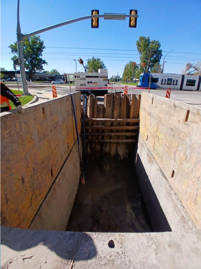
Well No. 18 Waterline – Bore Pit Excavation on the East Side of Trax
