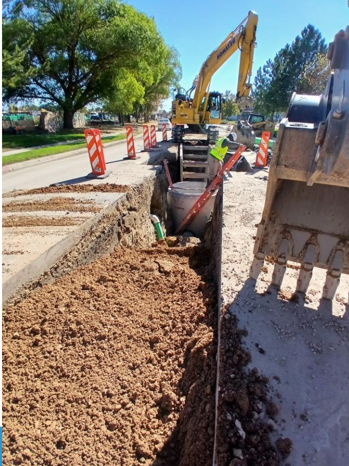
1950 W – Sewer Lateral Connection and Mainline Installation
