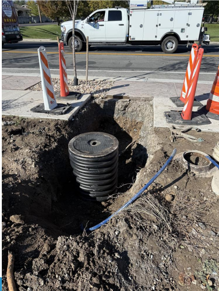
1" meter relocated out of sidewalk for new WVC park
