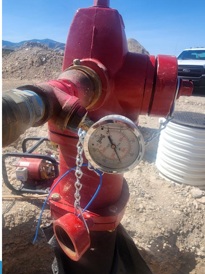
Pressure gauges for water main testing
