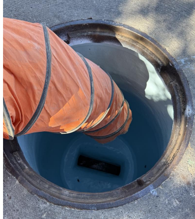
Manhole Rehabilitation Project – Ventilating manhole to protect worker's safety
