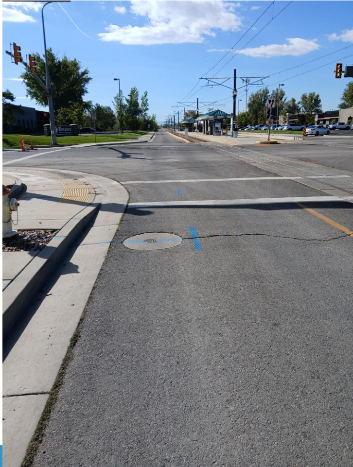
Marked location of 12" PVC water main
