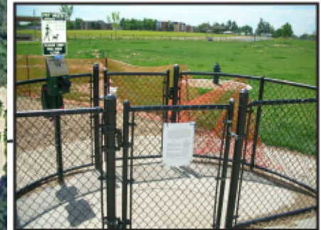
Double gate entry systems (4 Entries)
