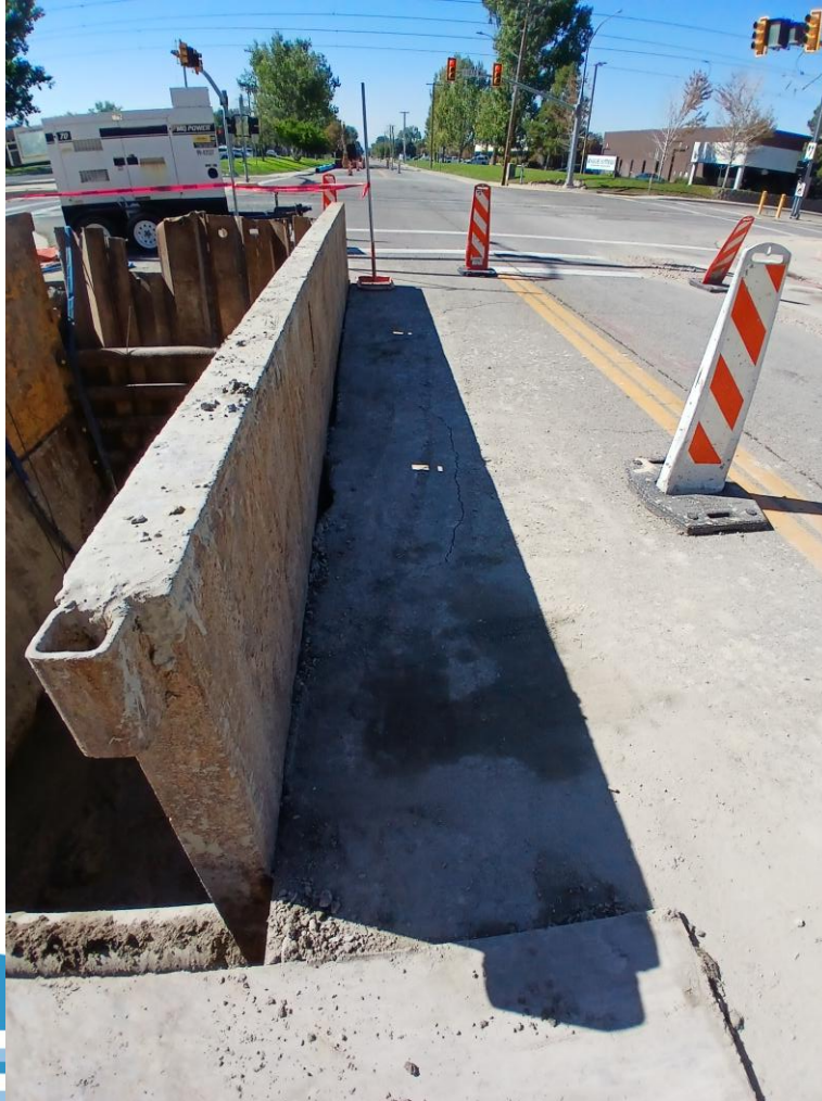
Roadway Cracking Due to Groundwater Induced Trench Collapse
