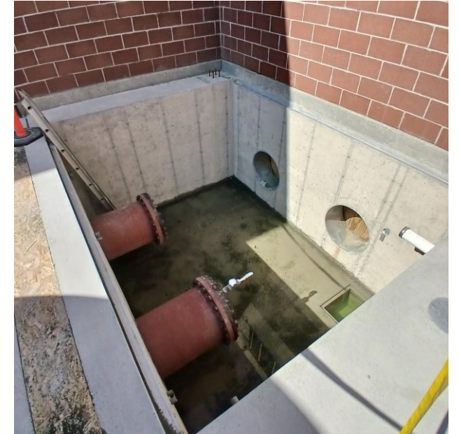
Anderson WTP Inlet & Outlet Piping
