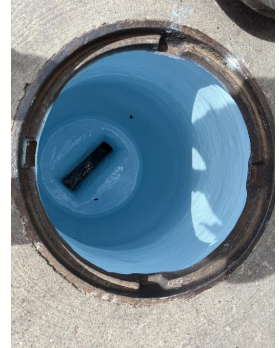
Manhole completed with Raven 405 Epoxy Liner system
