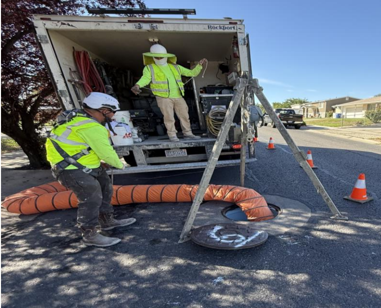
Pipeline Video Inspection employees preparing to add second epoxy liner coating to Manhole
