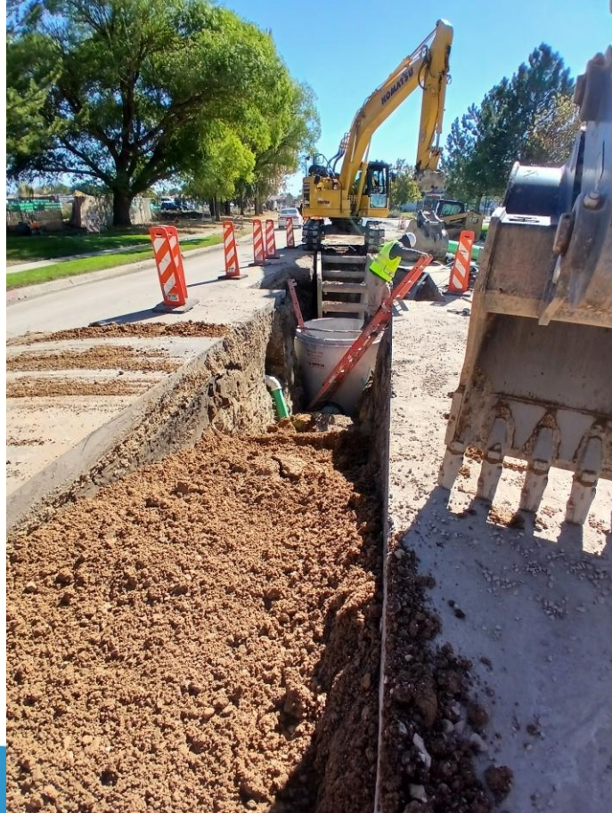
1950 W – Sewer Lateral Connection and Mainline Installation
