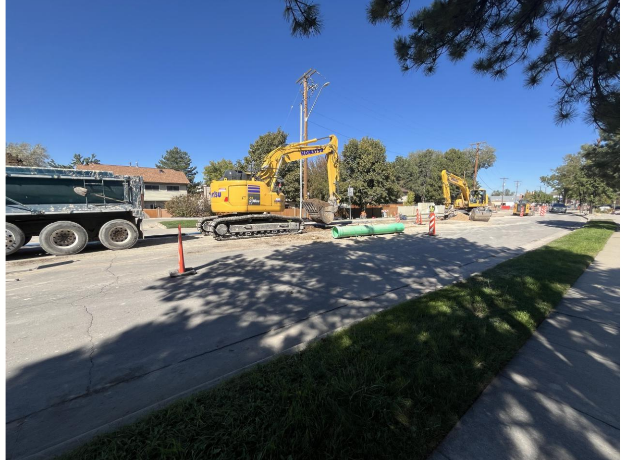
1950 W – Sewer Installation Setup
