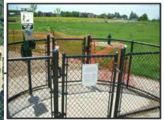
Double gate entry systems (4 Entries)
