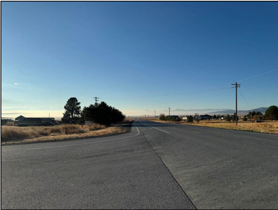
Southerly View of Highway 73 (NPA 7 on Left)
