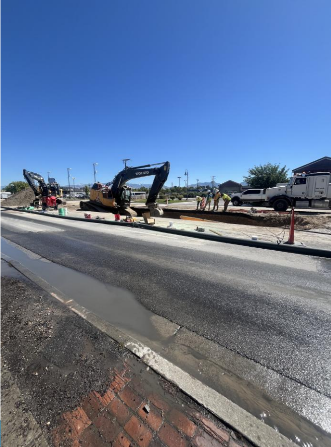
Redwood Road Sewer Installation
