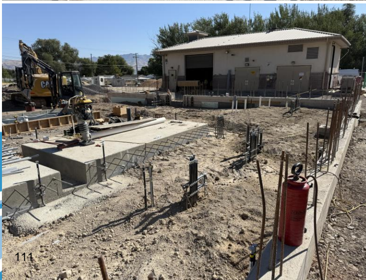
Electrical Conduit and Plumbing in Anderson WTP
