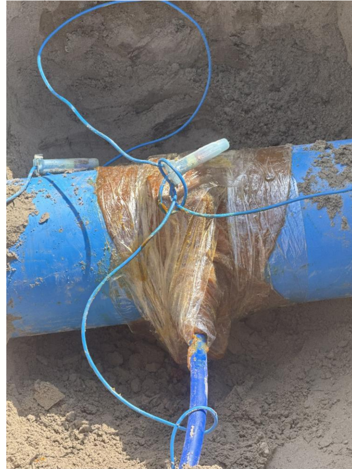
8" water line bend and water service wax wrapped
