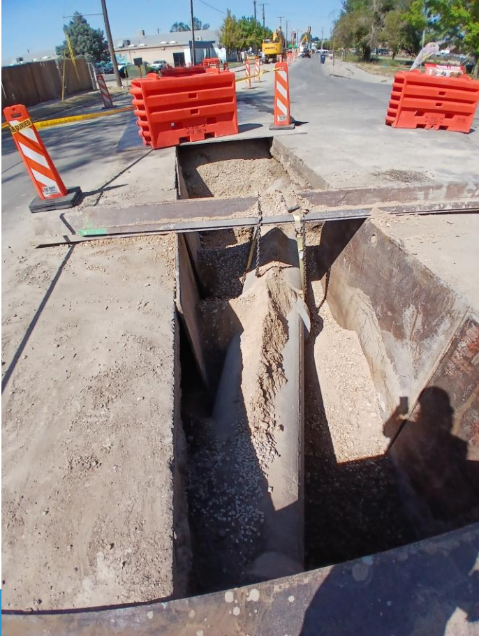
1950 W – Sewer Installation at Storm Drain Crossing
