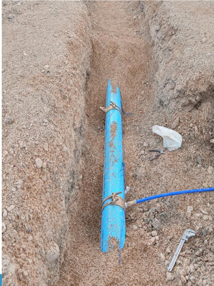
8" water main with \frac{3}{4} " water lateral connections
