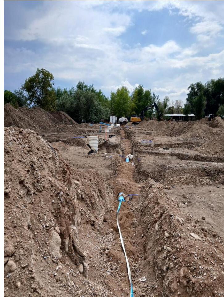
8" water main with \frac{3}{4} " water lateral connections
