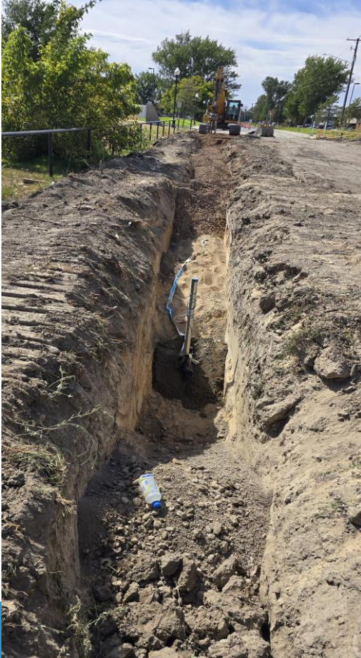
Well No. 18 Waterline – East Side Water Installation
