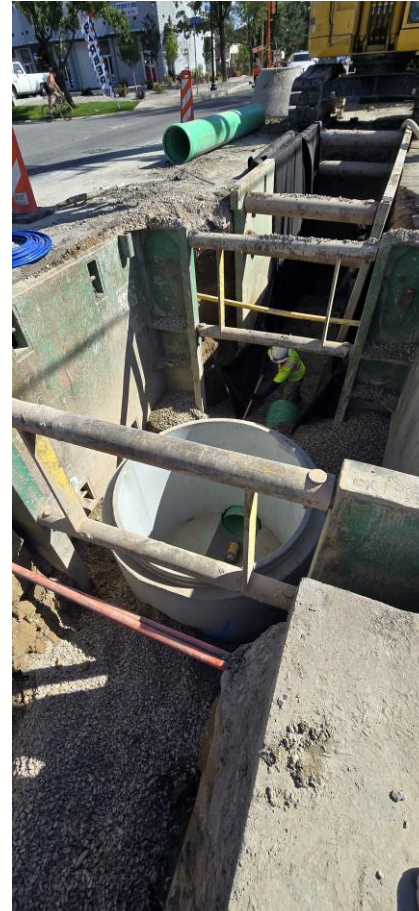
1950 W – Sewer Manhole Installation
