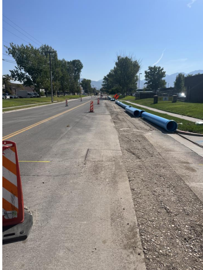
Well No. 18 Waterline – West Side Asphalt Removal
