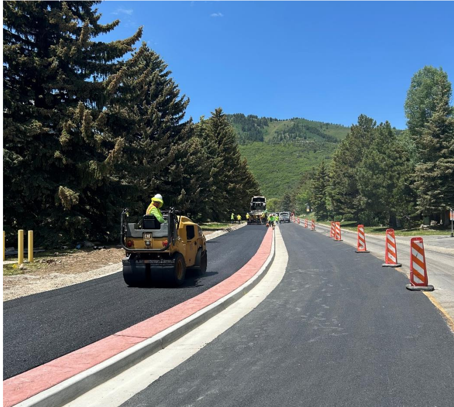
Figure 3 Phase 1 construction in progress on Thaynes Canyon Drive
