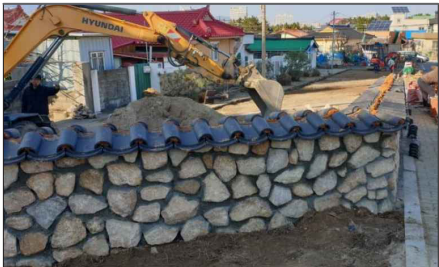
» Placing Adhesive Tile on Roof Tile (M), 3 Stage Tiling (F)
