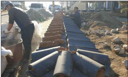
» Connecting Roof Tiles (M+F)
