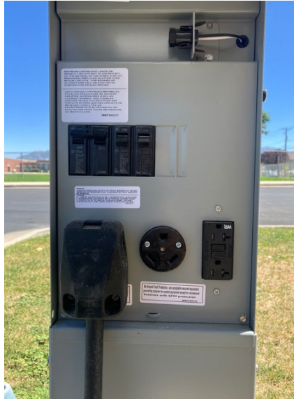
Requires a heavy duty plug and own power pedestal.
