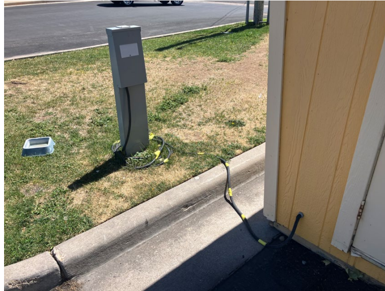
Requires a heavy-duty cord. Cord doesn't cross sidewalk or drive isle which is good. In way of mowing lawn maintenance/sprinklers. Power pedestal there specifically for business and no other use to city.
