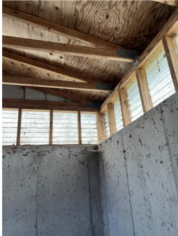
Photo 19 – Northeast Barn H1 Truss Attachment
