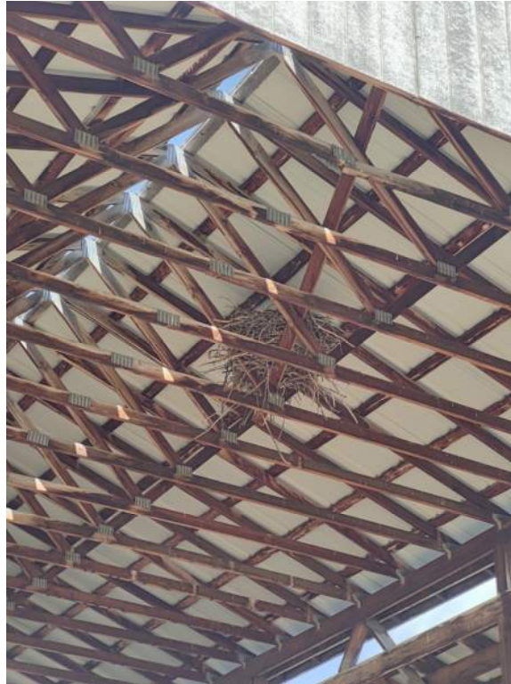
Photo 13 – Northwest Barn Broken Trusses
