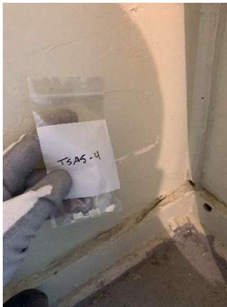
Photo #45 HA45: White "knock down" wall texture, not asbestos containing
