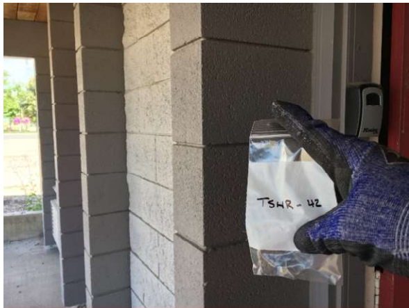
Photo #69 HA69: Exterior paint on block, not asbestos containing
