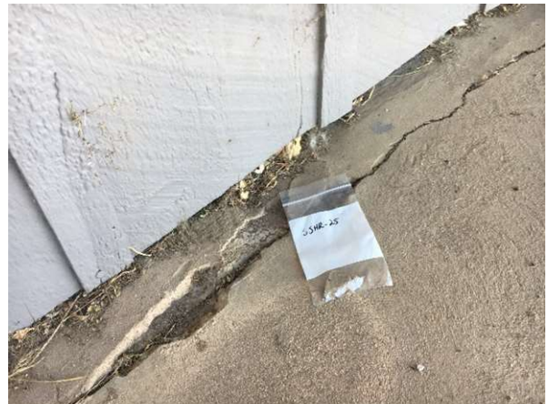
Photo #56 HA56: Concrete, not asbestos containing
