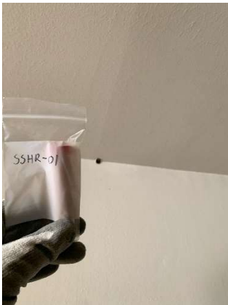
Photo #49 HA49: White gypsum board wall system, asbestos containing
