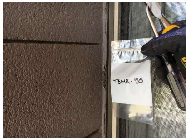
Photo #72 HA72: Window caulking, not asbestos containing
