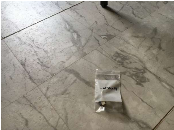
Photo #19 HA18: Light gray 12"x12" floor tile and mastic, not asbestos containing
