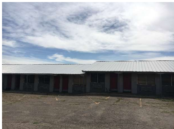
Photo #48 View of the single-story hotel rooms.
