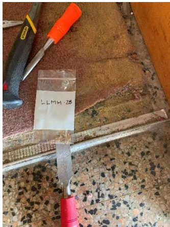
Photo #7 HA6: Carpet mastic, not asbestos containing
