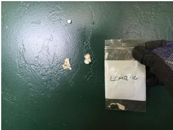
Photo #37 HA36: White wall texture, not asbestos containing
