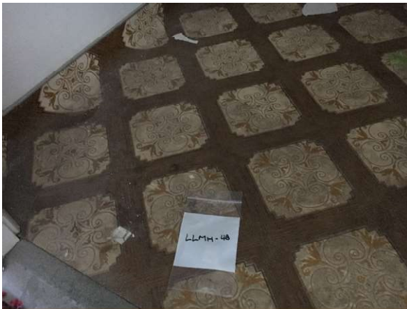
Photo #15 HA14: Brown 12"x12" vinyl tile with geometric pattern and mastic, asbestos containing
