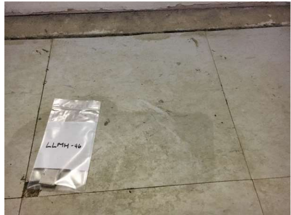
Photo #14 HA13: Gray 12"x12" floor tile and mastic and cementitious material, asbestos containing
