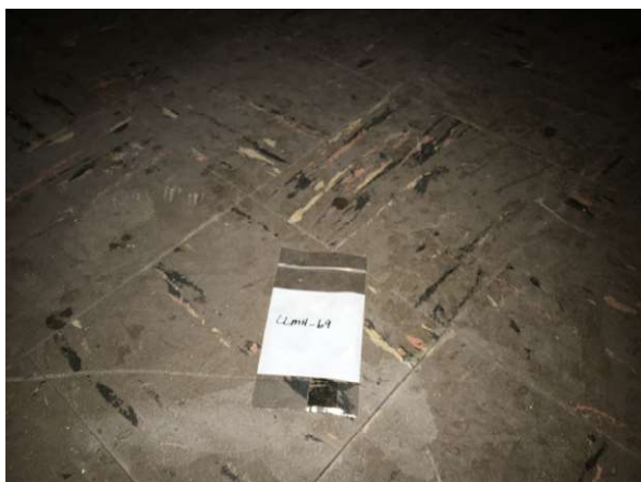
Photo #23 HA22: Brown 9"x9" floor tile with black, red, and white streaks and mastic, asbestos containing
