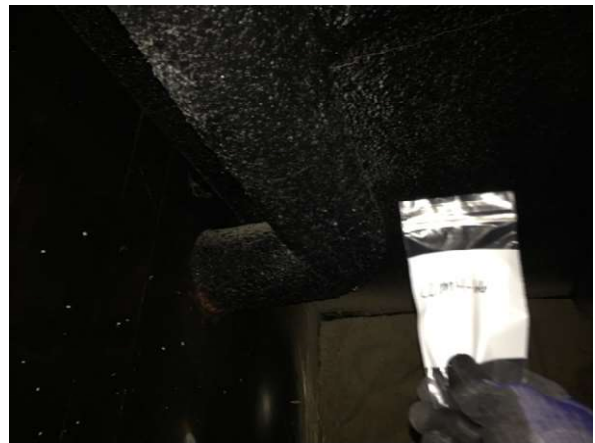
Photo #22 HA21: White mudded elbows, asbestos containing
