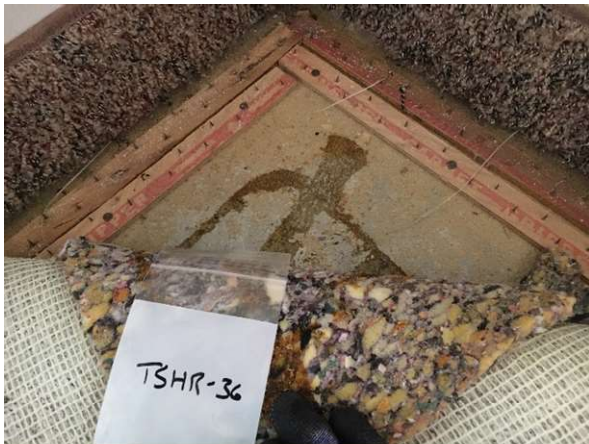
Photo #67 HA67: Carpet mastic, not asbestos containing
