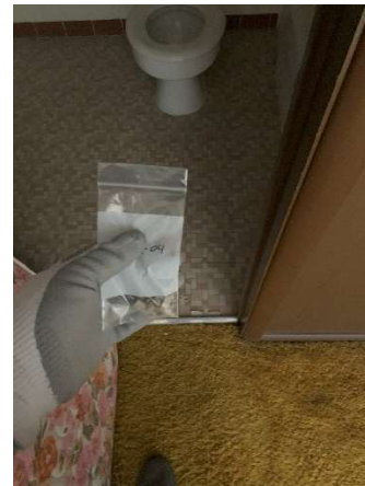
Photo #50 HA50: Thinset and grout, not asbestos containing
