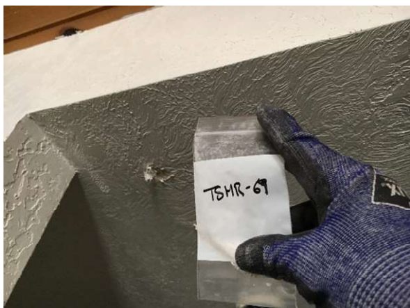
Photo #77 HA77: White swirl pattern ceiling texture, not asbestos containing
