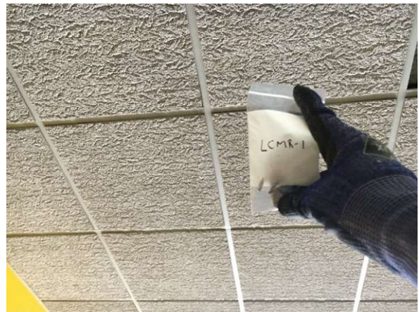
Photo #34 HA33: White 2'x2' rough texture ceiling tile, not asbestos containing
