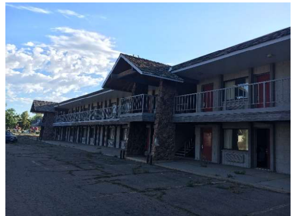
Photo #58 View of two-story hotel rooms.
