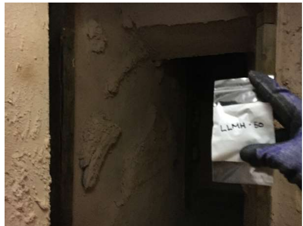
Photo #16 HA15: Cement coating on decorative cave, not asbestos containing
