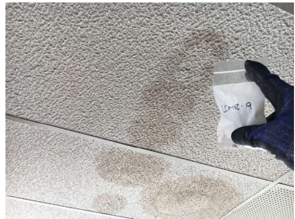
Photo #40 HA39: White 2'x4' ceiling tile with bumpy texture, not asbestos containing
