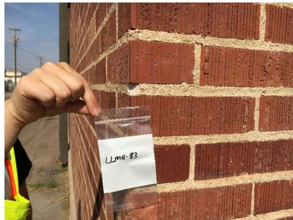
Photo #28 HA27: Mortar, not asbestos containing (incorrect sample number in photo)
