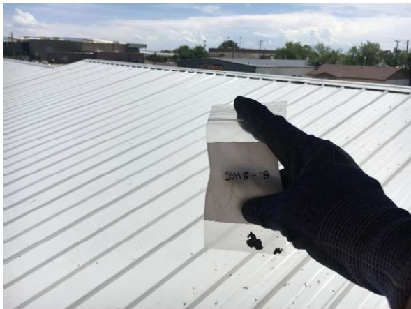
Photo #57 HA57: Tar paper roofing, not asbestos containing
