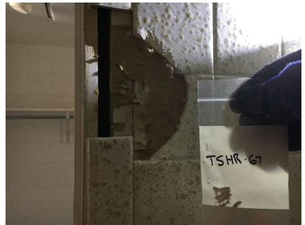
Photo #76 HA76: Grout and adhesive, not asbestos containing
