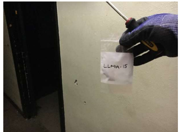
Photo #4 HA3: Plaster walls and ceilings, not asbestos containing
