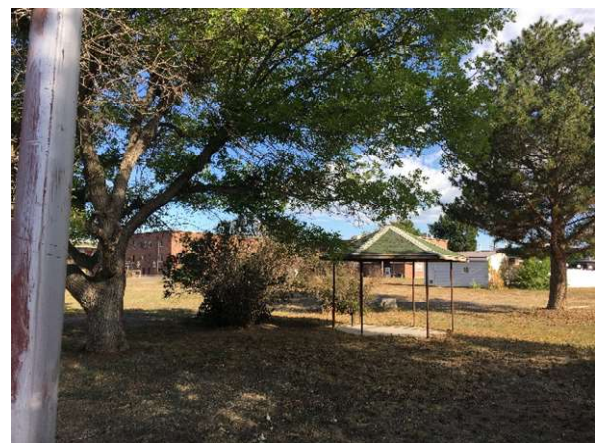
Photo #78 View of pump house in background no suspect materials identified.
