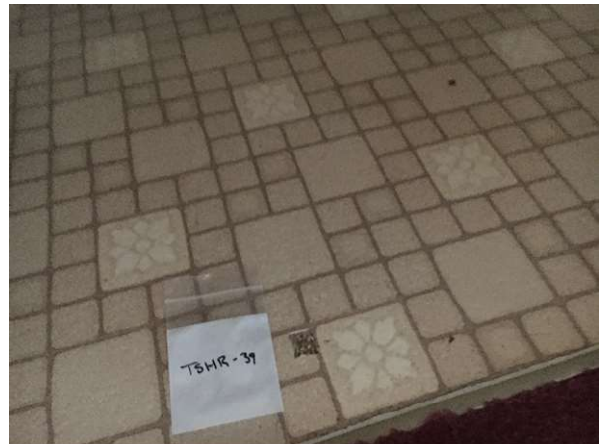
Photo #68 HA68: Thinset and grout, not asbestos containing
