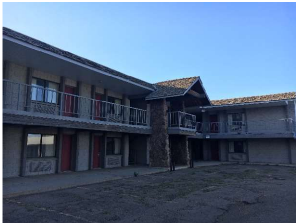
Photo #75 HA75: Roof tar paper (under shingles), not asbestos containing
