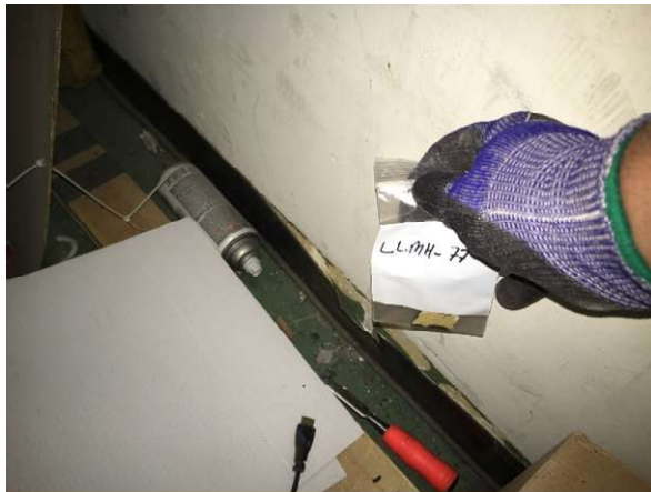
Photo #27 HA26: Tan cove base adhesive, not asbestos containing
