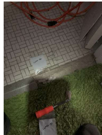
Photo #10 HA9: Thinset and grout, not asbestos containing
