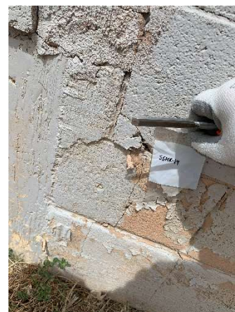
Photo #54 HA54: Paint on block, not asbestos containing
