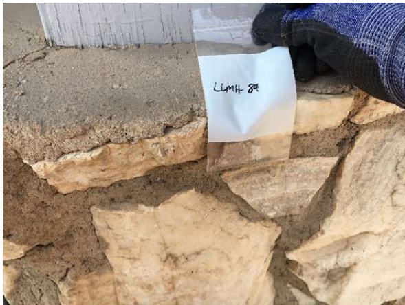
Photo #31 HA30: Decorative rock formation mortar, not asbestos containing
