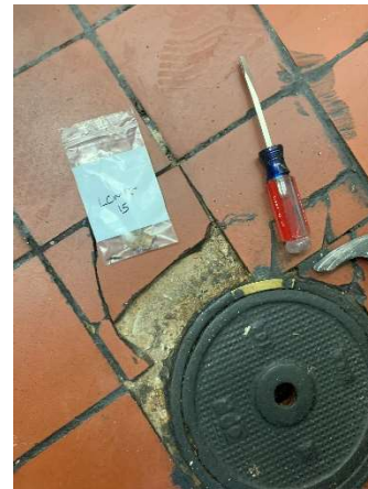
Photo #38 HA37: Thinset and grout, not asbestos containing
