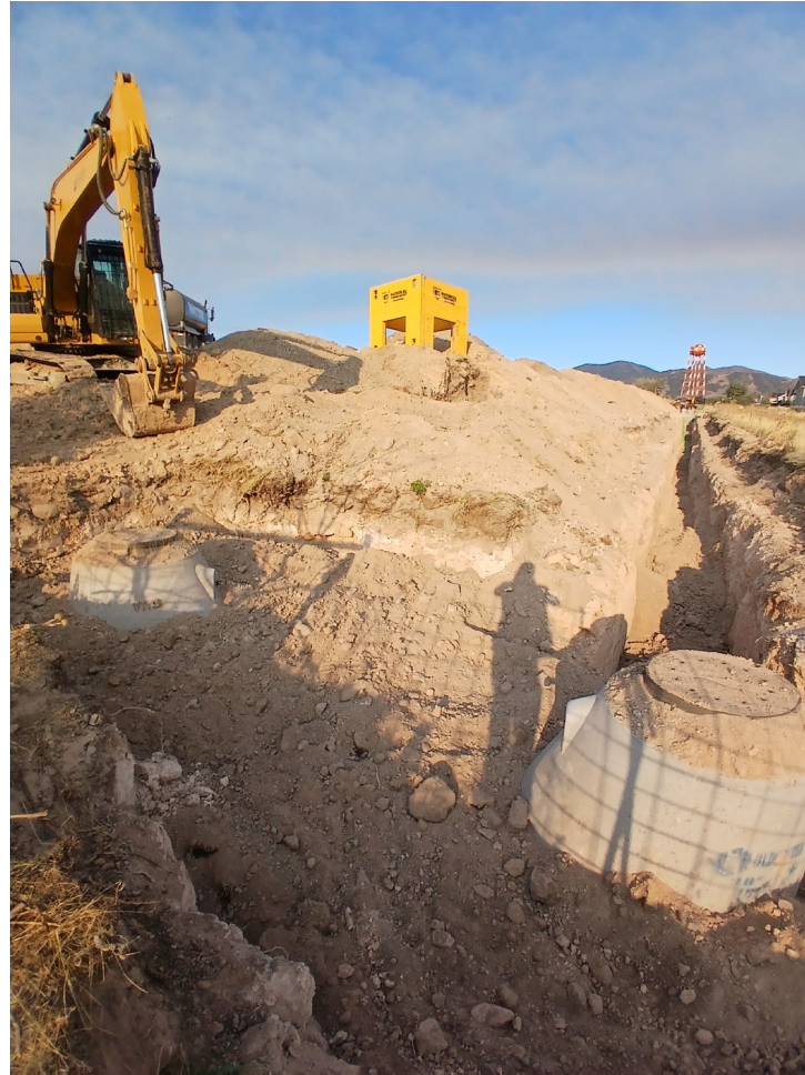
Sewer manholes and lateral trench
