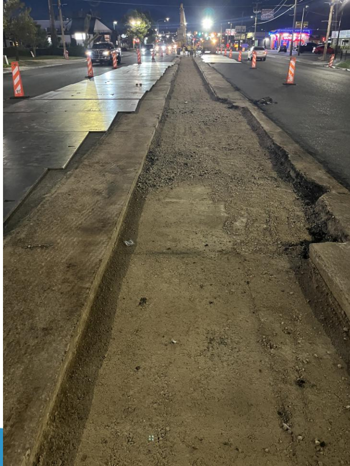
3500 South Backfill Placement
