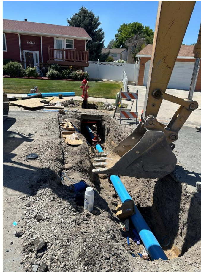
Cherrywood Waterline – GHID crew installing main, valve and hydrant for cul-de-sac
