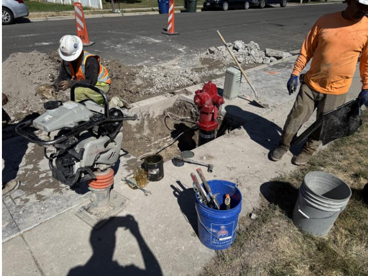
PNL Construction Installing Hydrant
