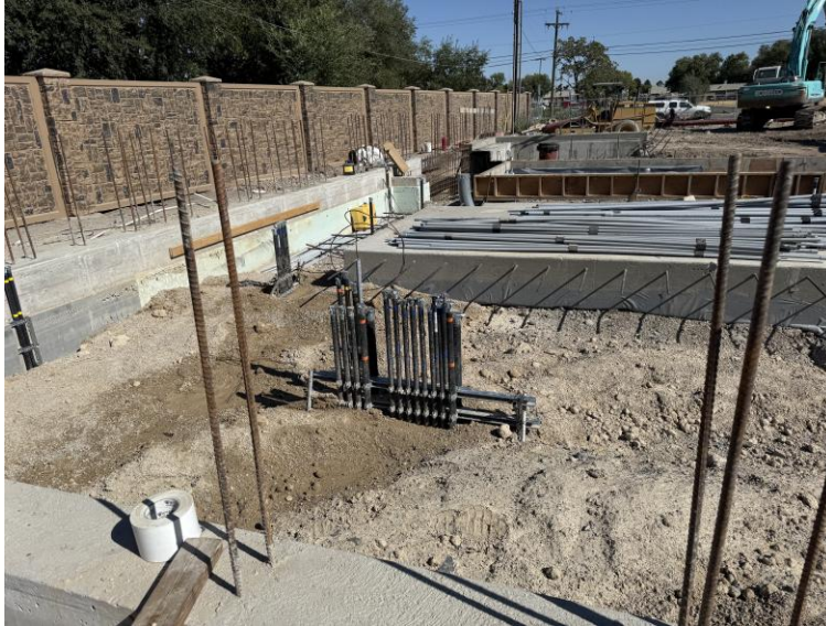
Electrical conduit installed in future Southwest corner of Anderson WTP
