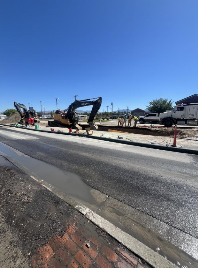
Redwood Road Sewer Installation
