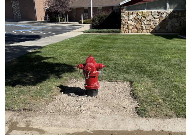
Hydrant Installed Prior to Concrete Pad Being Poured
