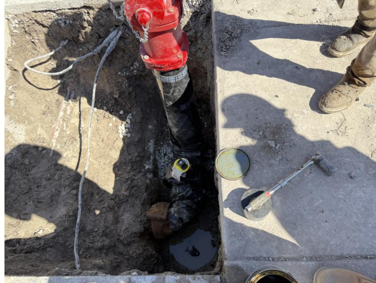
Newly Installed Hydrant and Valve
