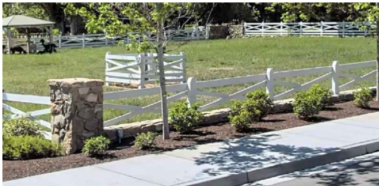
LOW STONE WALL WITH FENCE ON TOP
