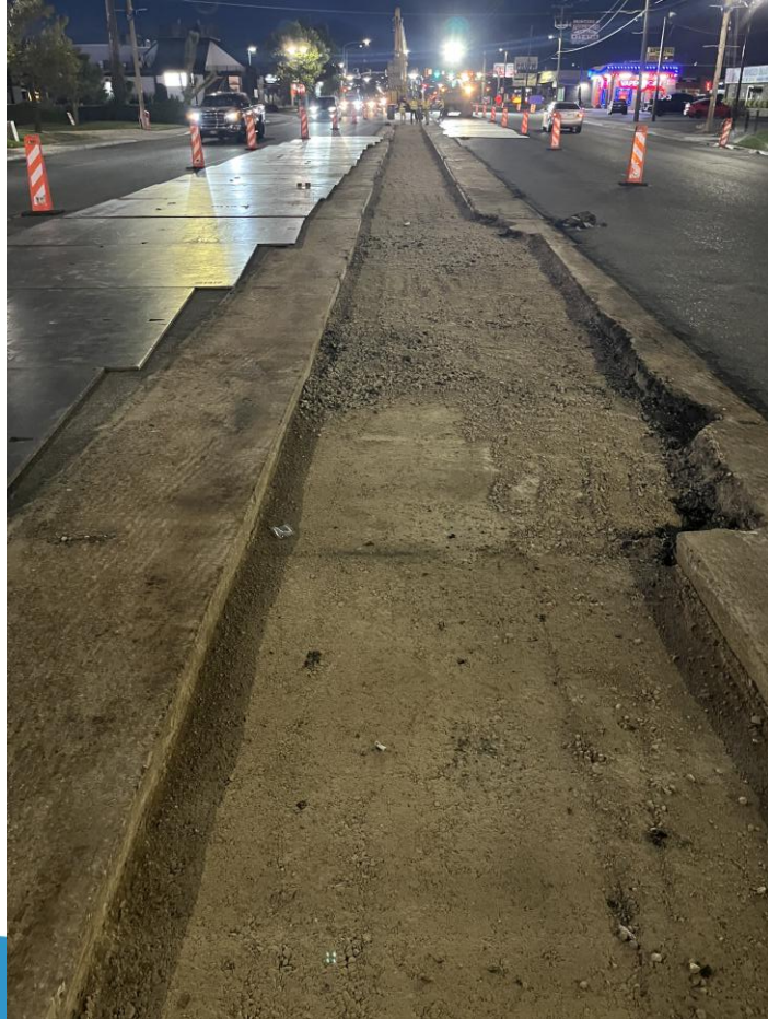
3500 South Backfill Placement
