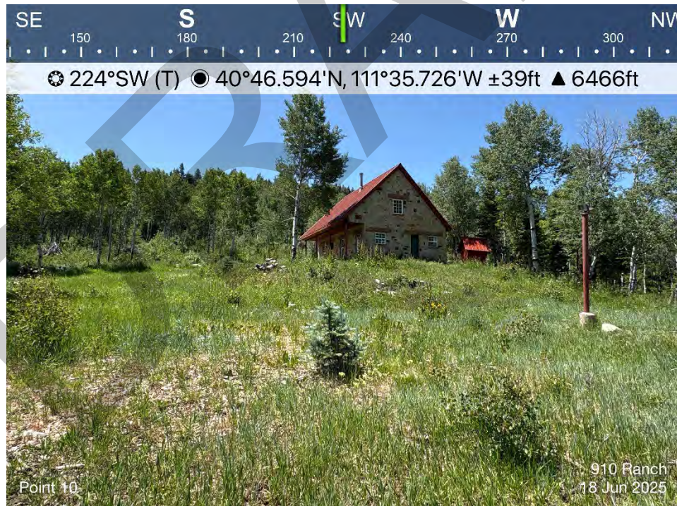
Point 10. Stone structure
