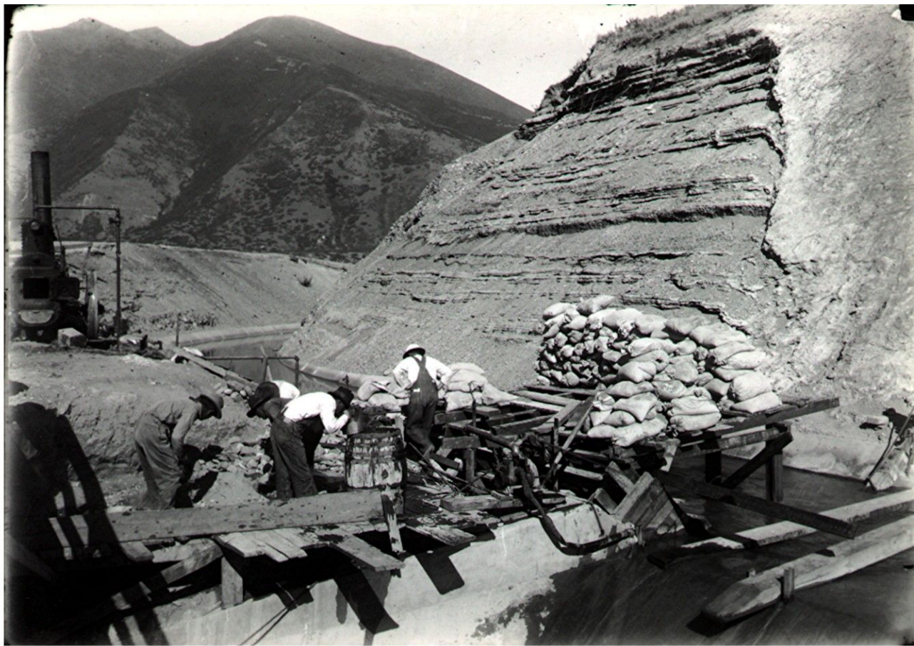
Strawberry Power Canal: Culvert During Construction of Wasteway of the Forebay
