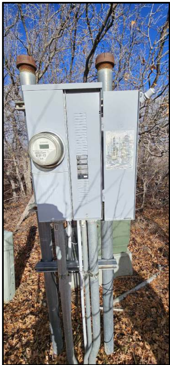
PHOTO 1: VIEW OF THE EXISTING ELECTRICAL PANEL, METER, AND SWITCH.
