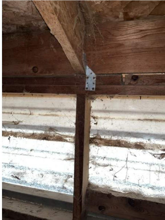
Photo 6 – Southwest Barn Joist H2.5 Attachment
