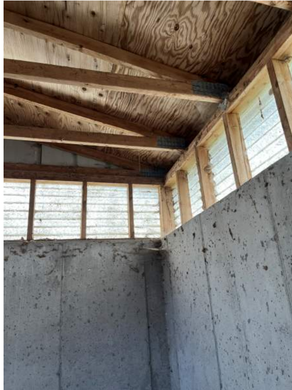
Photo 19 – Northeast Barn H1 Truss Attachment
