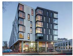
The ground level is differentiated with larger areas of transparency from the levels above utilizing a mix of materials, opacities, and facade articulation
