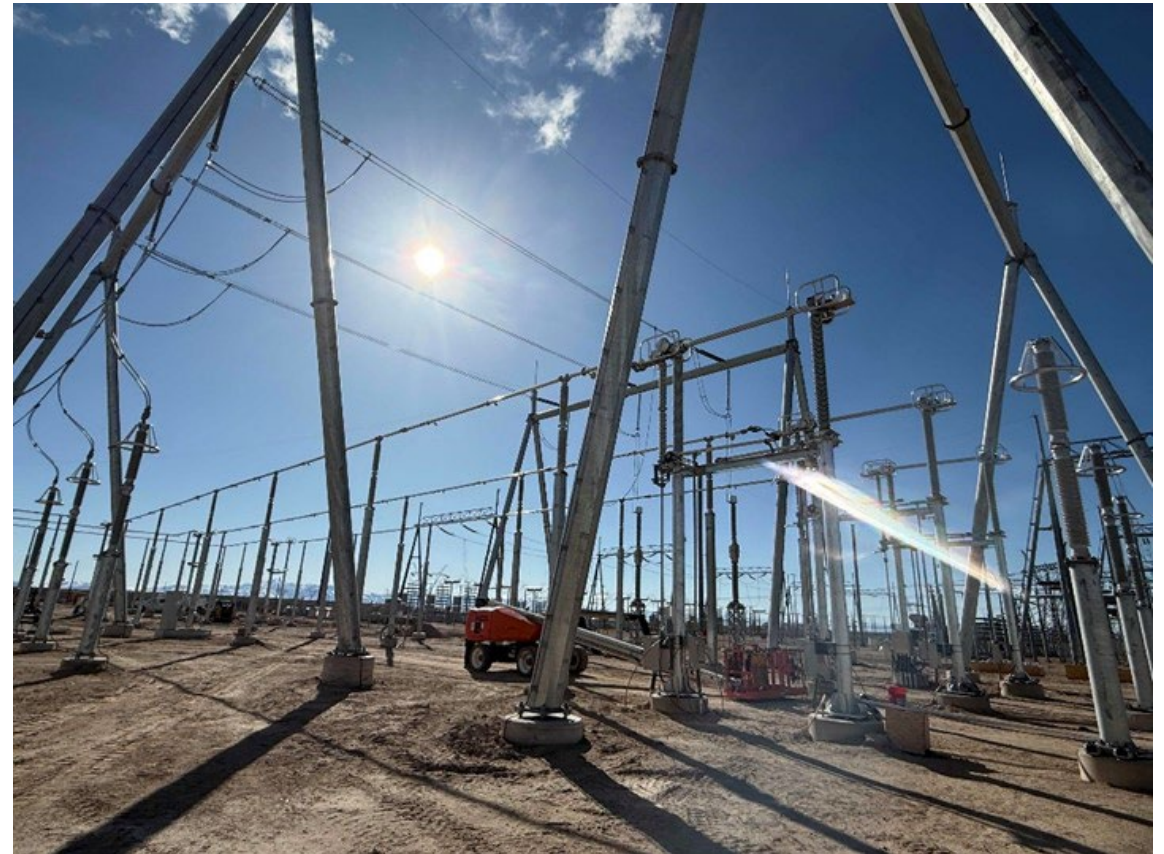
345 kV OH conductor
