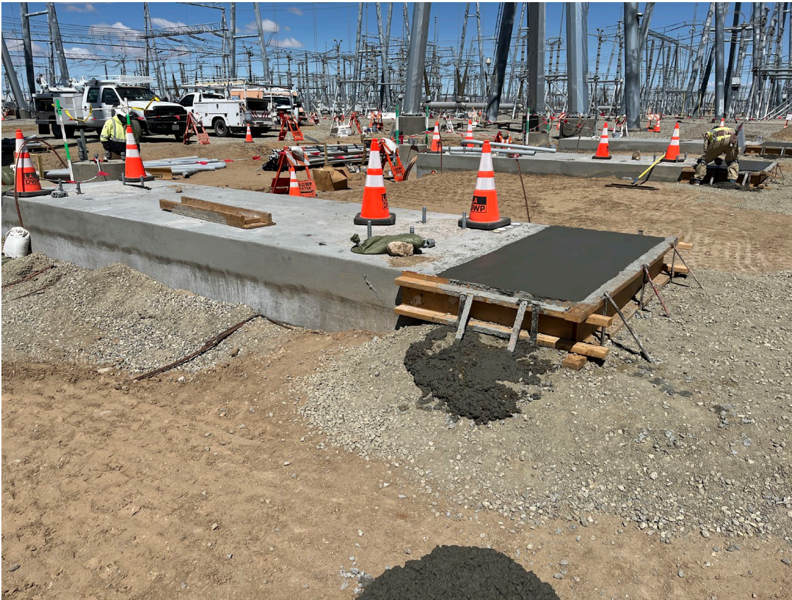
Line Side Disconnect Foundations Curing and Operator Pads
