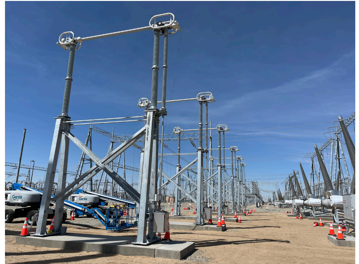
Bus Side Disconnects Support Steel & Switch Installed
